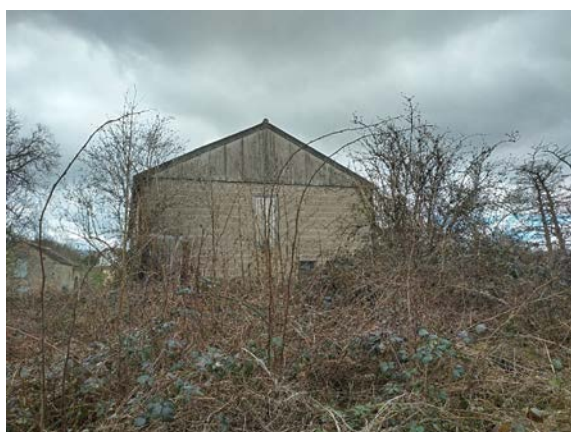
Photo 13: T17 and T18 from north west
