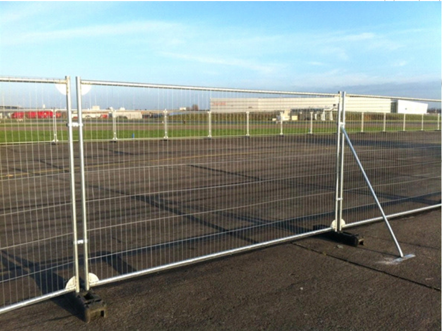
Inset 1: Tree protection fencing
