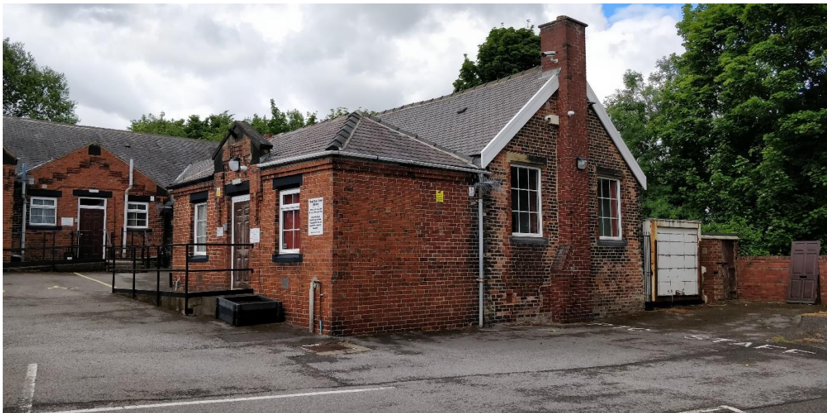
Existing Site Photo
