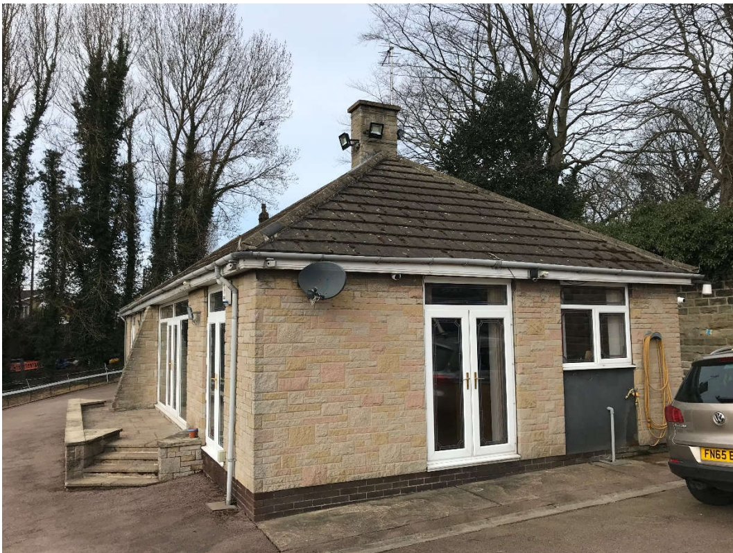
Fig 04. South and East Elevation of existing bungalow.
