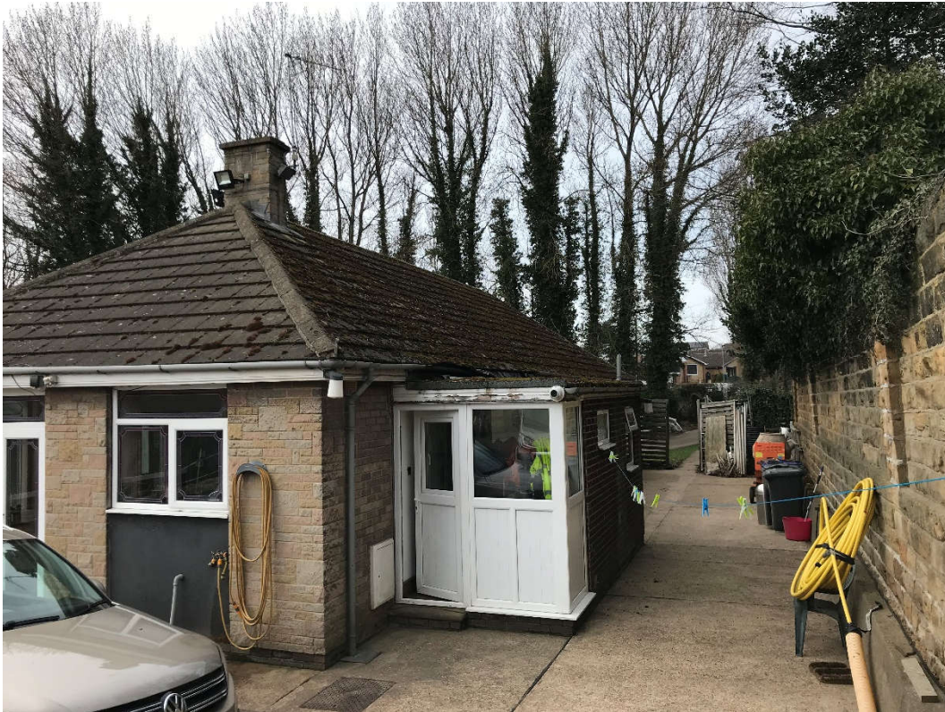
Fig 05. Rear North Elevation showing proch and high boundary wall to north (right).
