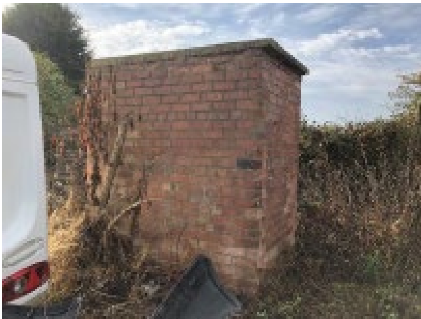
Brick – built toilet block
