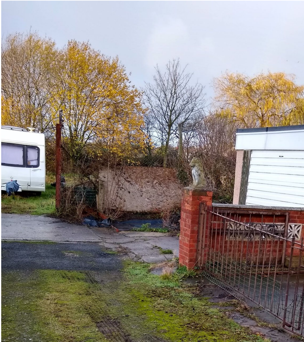
End of path / site entrance
