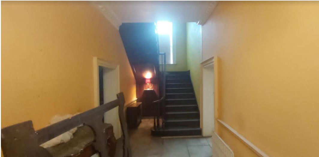
Fig 26 Central entrance hall and main stairs with service passage beneath half landing
