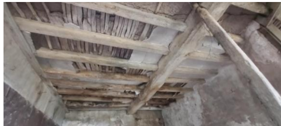
Fig 44 Lath and plaster ceiling to stall
