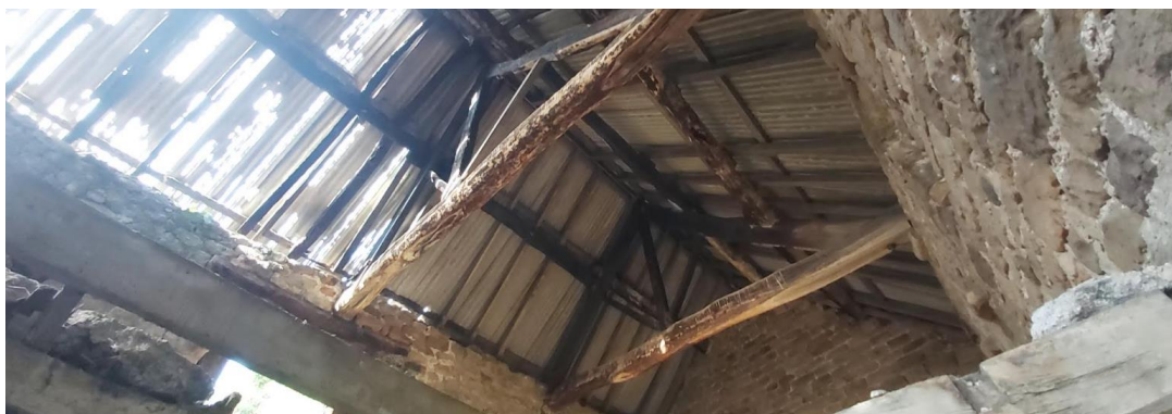
Fig 69 King post roof structure
