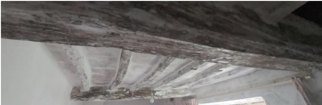
Fig 52 Historic, principal timber beams and joists in first floor, right hand, front room
