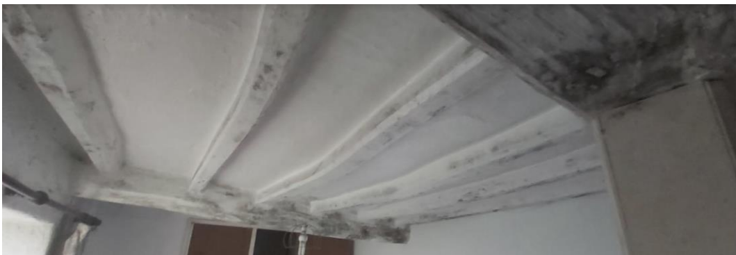
Fig 53 Historic, principal timber beams and joists in first floor, right hand, rear room
