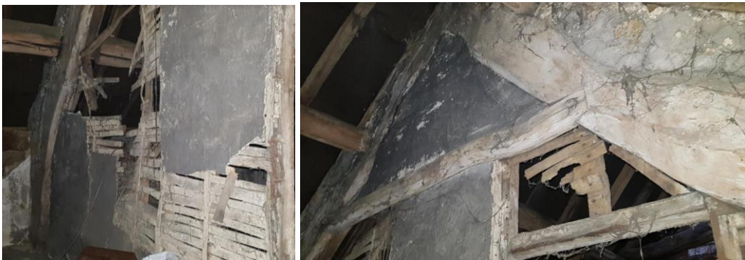
Fig 48 Rear cruck blade & partition Fig 49 Upper blades with tie beam and door opening
