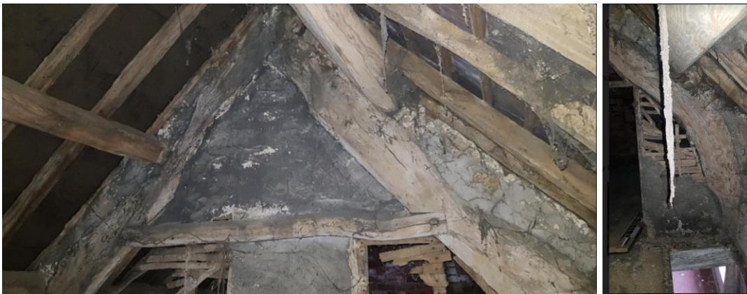
Fig 50 Upper crucks with wattle and daub partition and tie beam below Fig 51 Front blade
