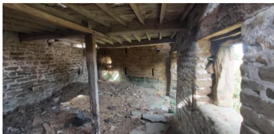
Fig 67 Latts to ceiling
