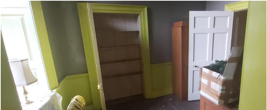
Fig 22 Panelled doors, fitted cupboards, panelling and window shutters in ff, central room
