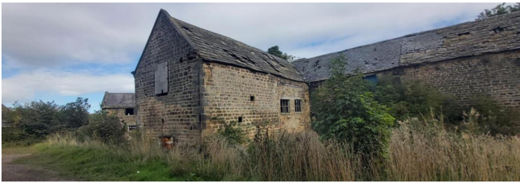
Fig 41 Rear elevation of cart shed/stables to right, attached gable dairy to left
