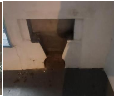
Fig 21 Evidence of former fireplace in south, attic gable
