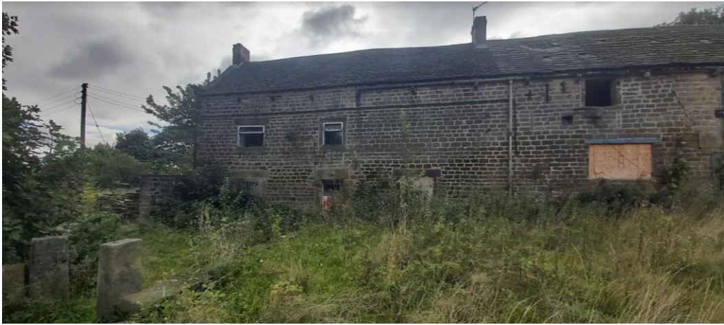
Fig 47 Rear elevation of Farm Cottage with stone gate posts and walled garden
