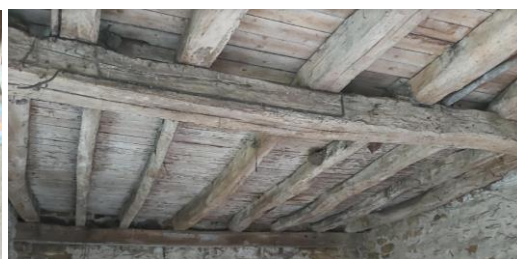
Fig 63 Historic roof structure
