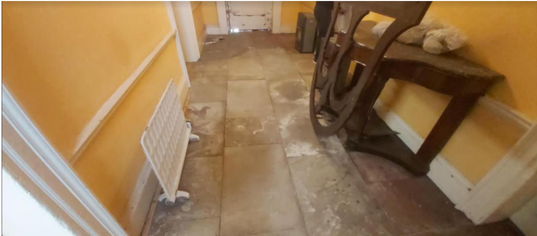
Fig 27 Stone flagged, ground floor hall with dado rail from rear to front door
