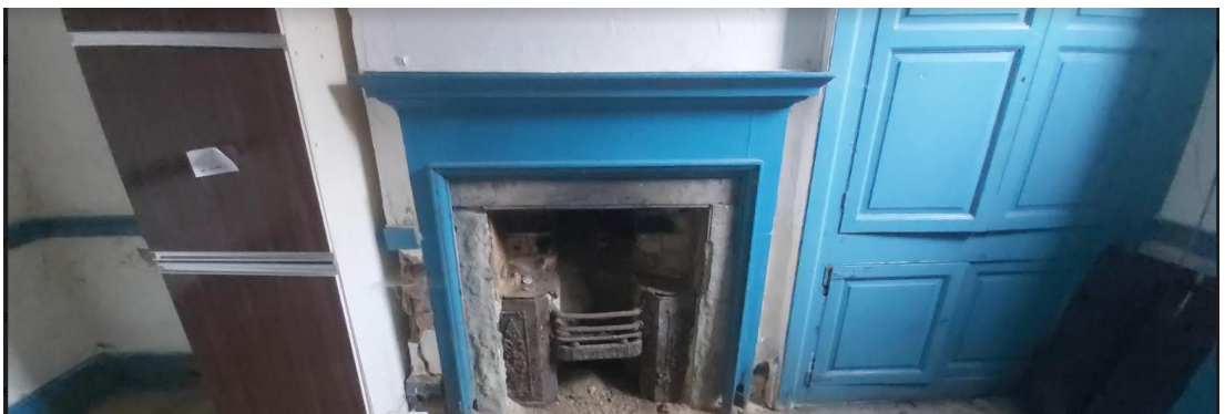
Fig 23 Fireplace, fitted cupboard, dado and skirting to ground floor, rear service room
