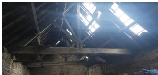
Fig 58 Concrete lining and modern first floor Fig 59 King post trusses within dairy
