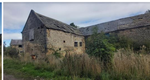
Fig 57 Principal dairy southern elevation
