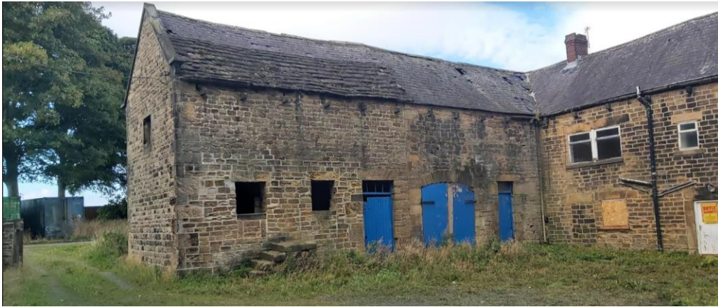
Fig 40 Cart shed and stables with mounting block attached to Farm Cottage
