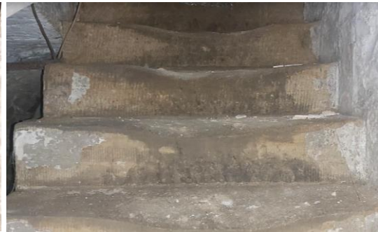
Fig 13 Cellar steps, dished with wear
