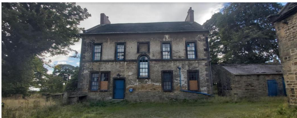
Fig 7 Rear, north facing elevation
