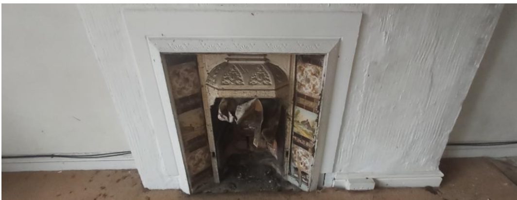
Fig 54 Victorian fireplace in first floor, left hand room
