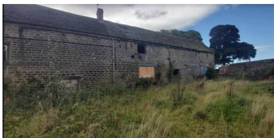
Fig 56 Principal dairy north elevation
