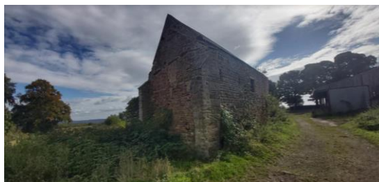
Fig 68 Approach from north-west
