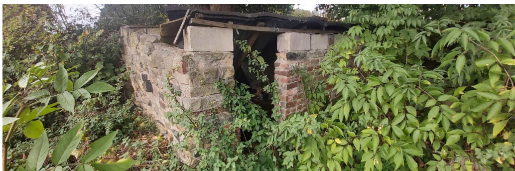
Fig 55 Remains of structure on land to north-east of Farm Cottage
