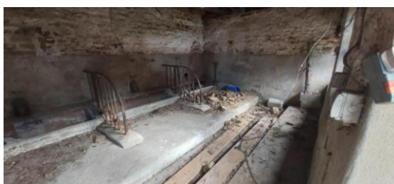
Fig 62 Cement lined ground floor & lime above
