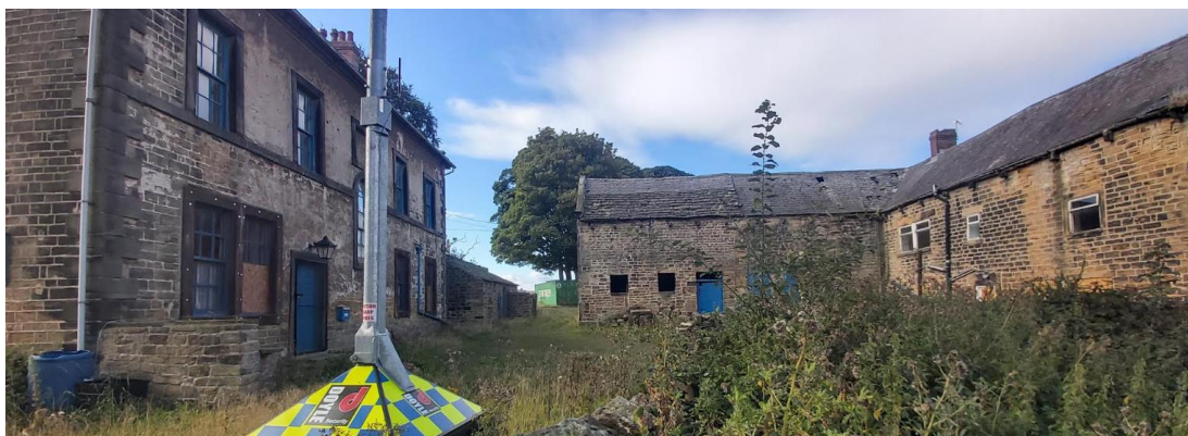
Fig 37 Direct, visual relationship between house, cart shed and Farm Cottage
