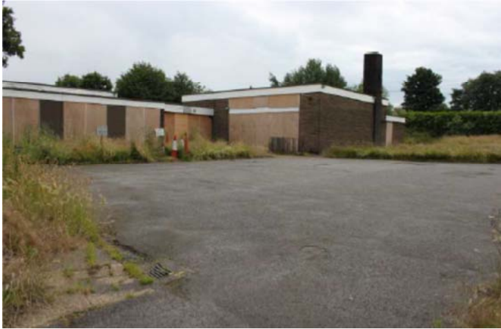
Existing buildings on site
