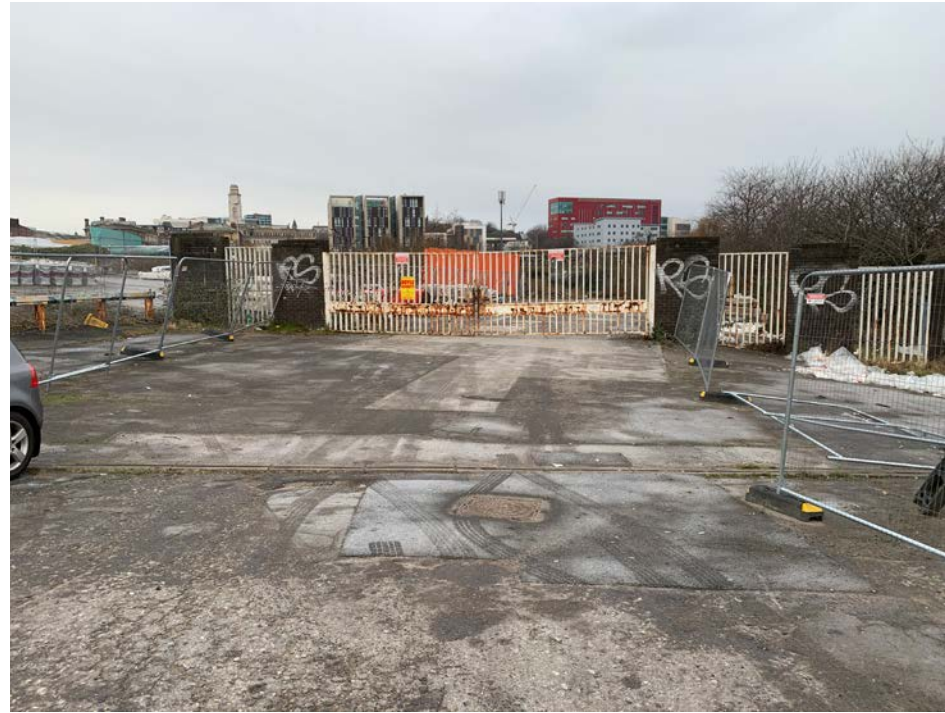
View looking west from Harborough Hill Road
