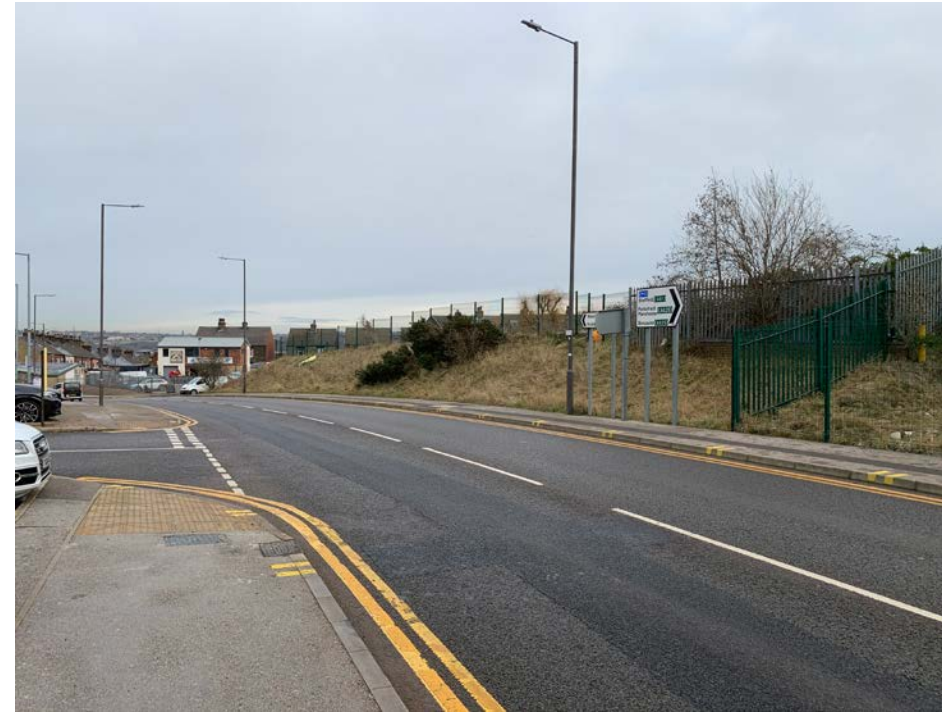
View of banking facing Schwäbisch Gmünd Way
