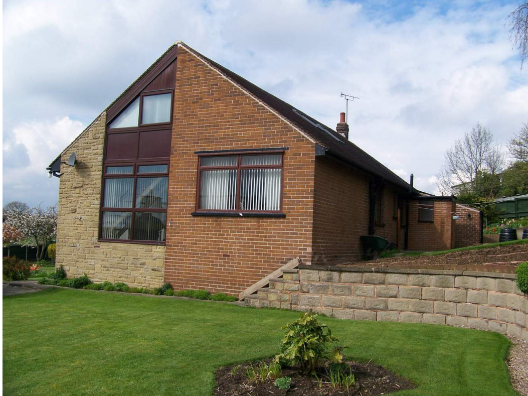
Photo 3 East facing gable elevation onto which the extension is to be added. The level lawn area is set down from the floor level land only minimal excavation will be required. The general slope of the land and the essential single storey nature of the building reduce any overshadowing of neighbouring properties.
