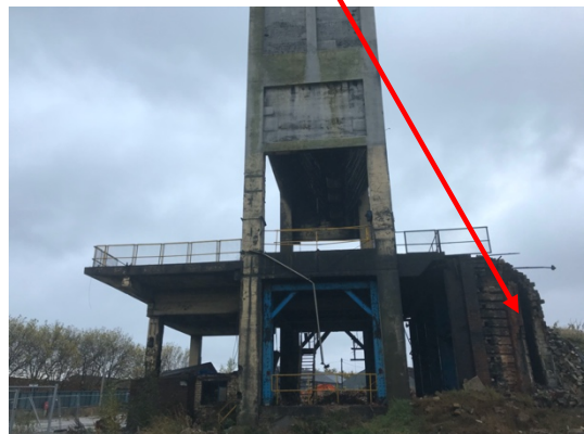
Image 26: Collapsed brickwork
