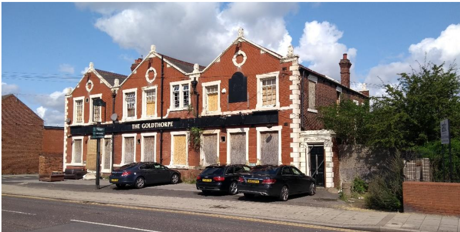
View of main façade to Doncaster Road
