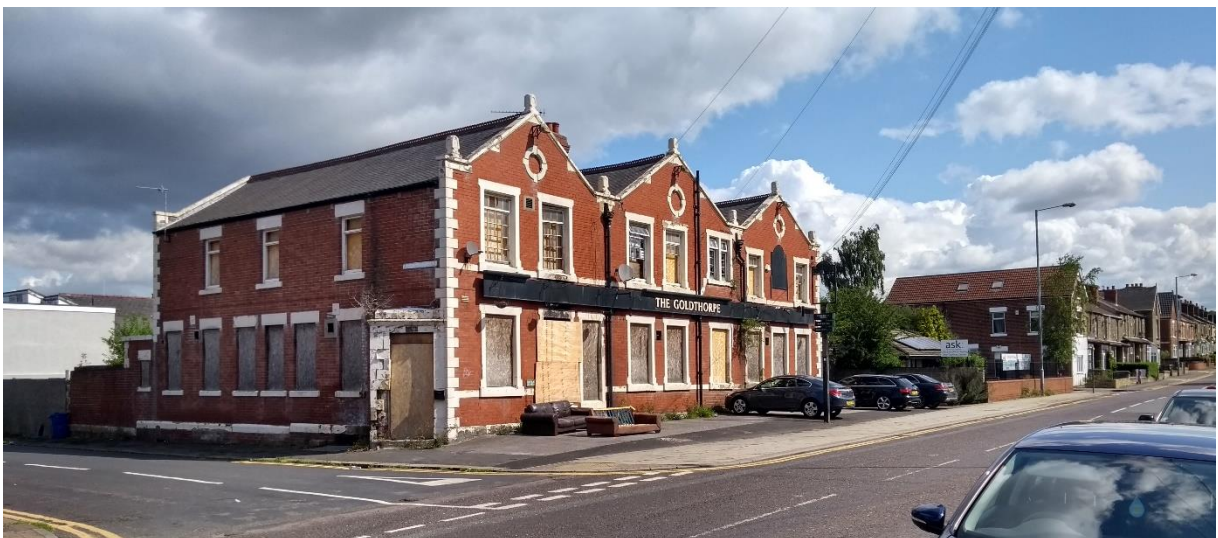
South-West view of the Goldthorpe Hotel building from Hamilton Road junction
