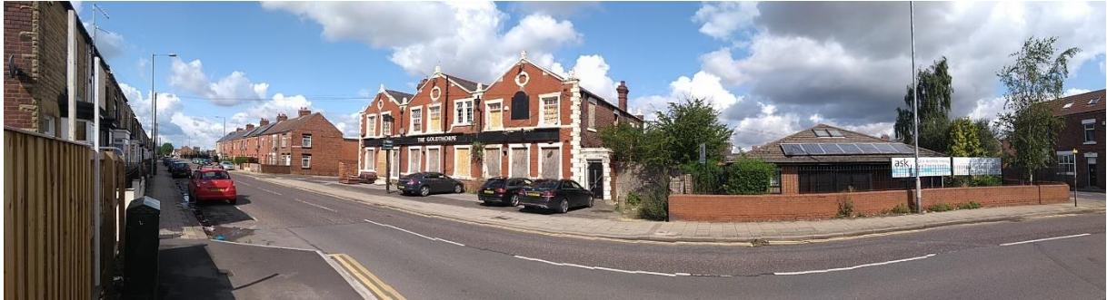
South-East view of the Goldthorpe Hotel building from Doncaster Road
