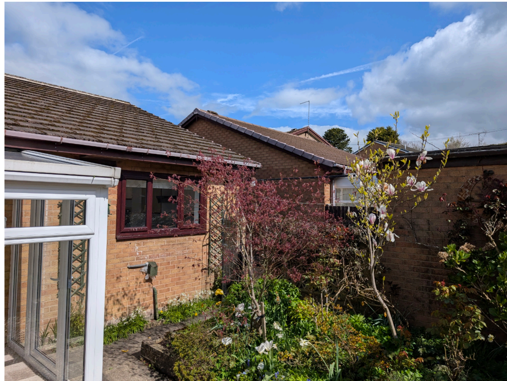
2604 - 28 Windermere Rd, Penistone, Sheffield, S36 8HL Rear of neighbouring properties to the East
