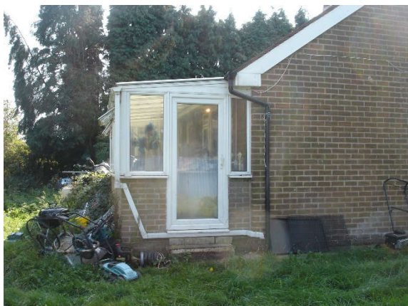
Fig 05. Gable north and rear lean-to
