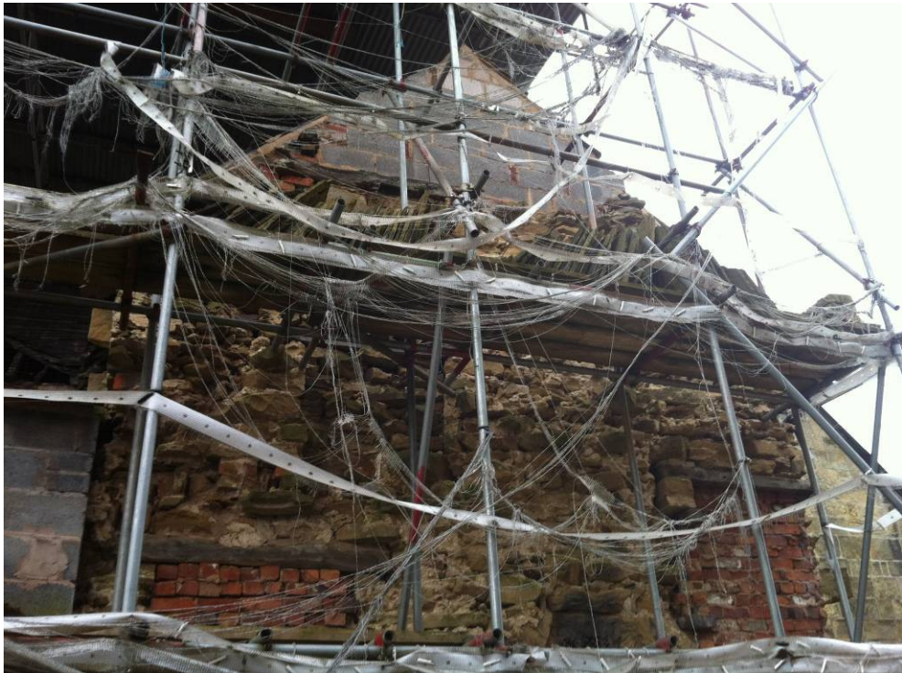
4. Upper gable wall of rear offshot.
