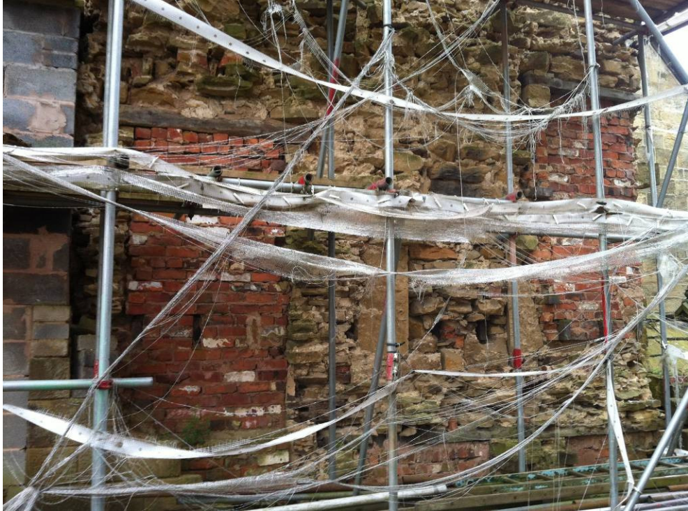
3. North elevation of rear offshot (through scaffolding).
