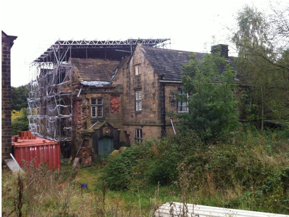
View of north elevation of Worsbrough Hall (October 2012) with protective scaffolding.
