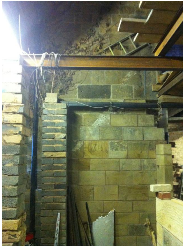
8. West elevation of external wall adjacent D1.
