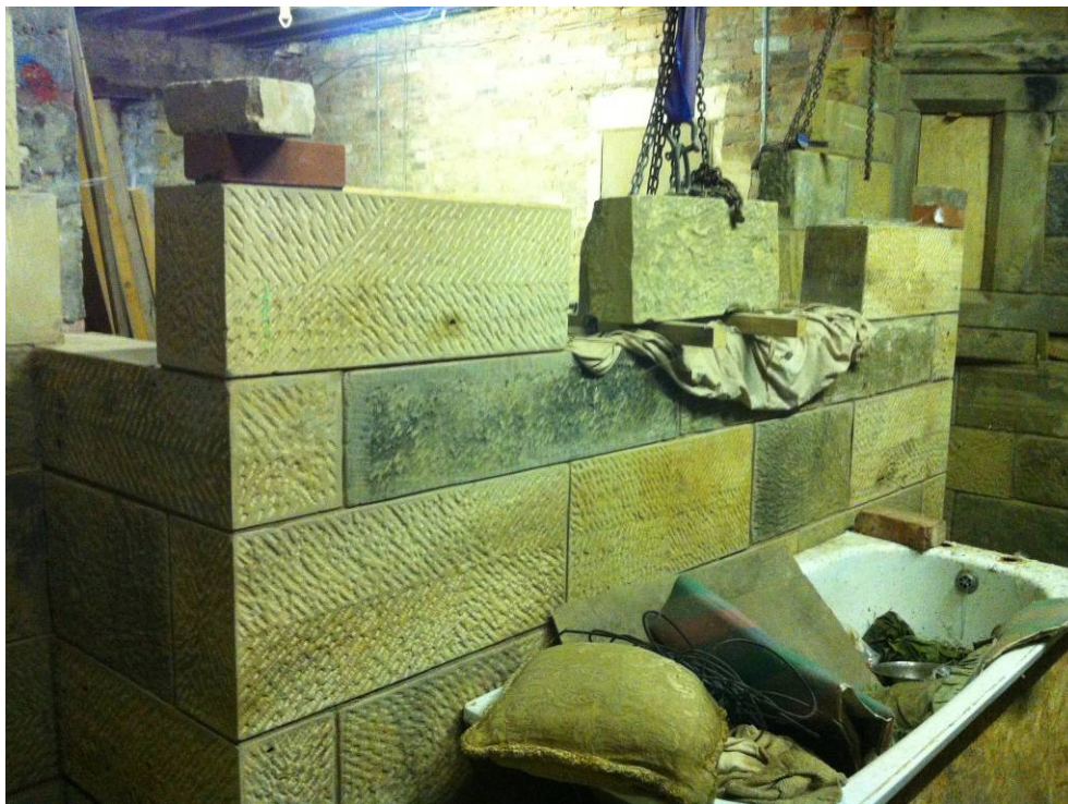
6. External view of chimney stack under construction.
