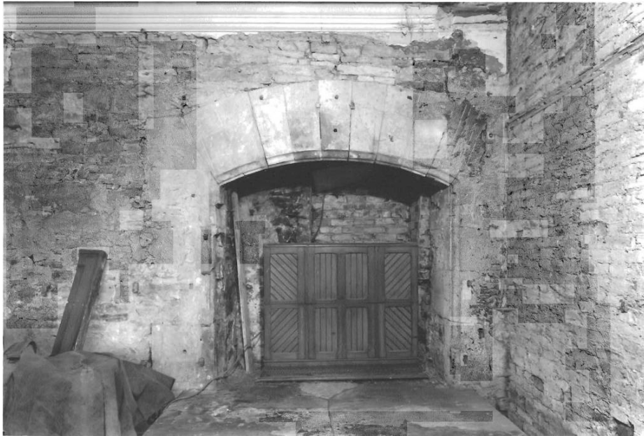
View of original ground floor fireplace to be reinstated.
