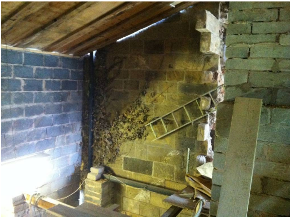
12. West elevation of external wall adjacent D1 – first floor level
