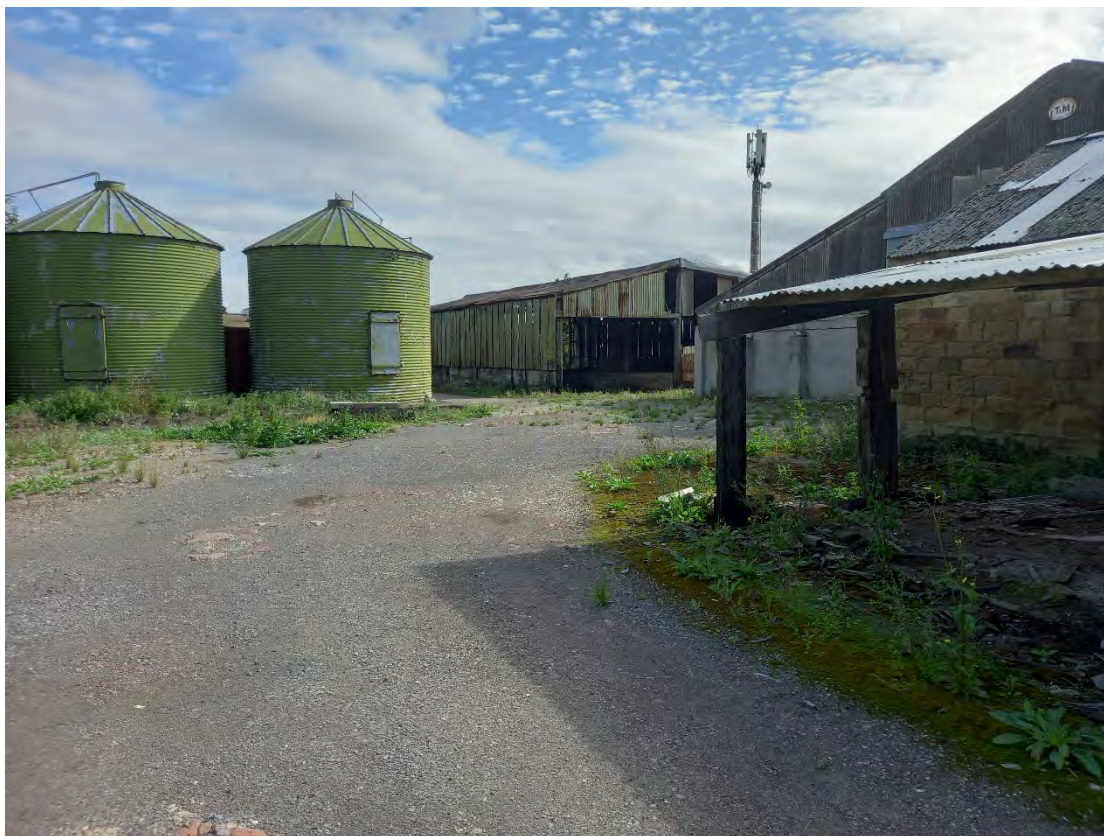
Plate 6. Modern agricultural buildings and silos on the south-western side of the study site, looking north-east
