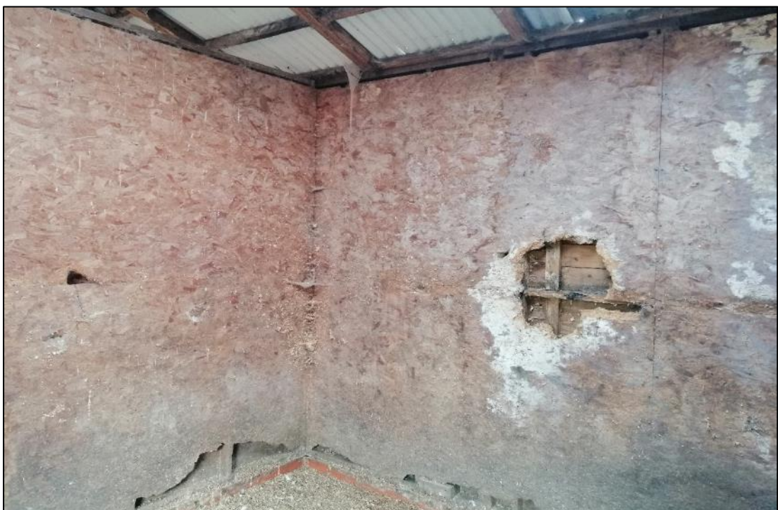
Plate 5. Inside of a stable compartment showing damaged sterling board
