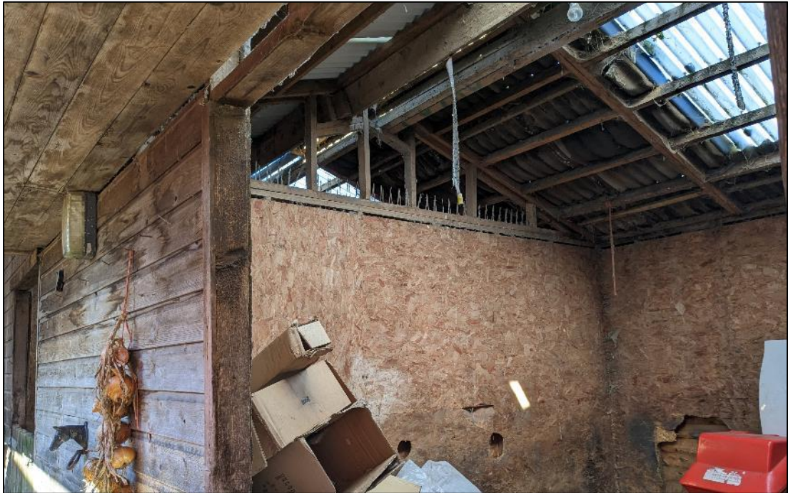
Plate 5. Inside of a stable compartment showing damaged sterling board
