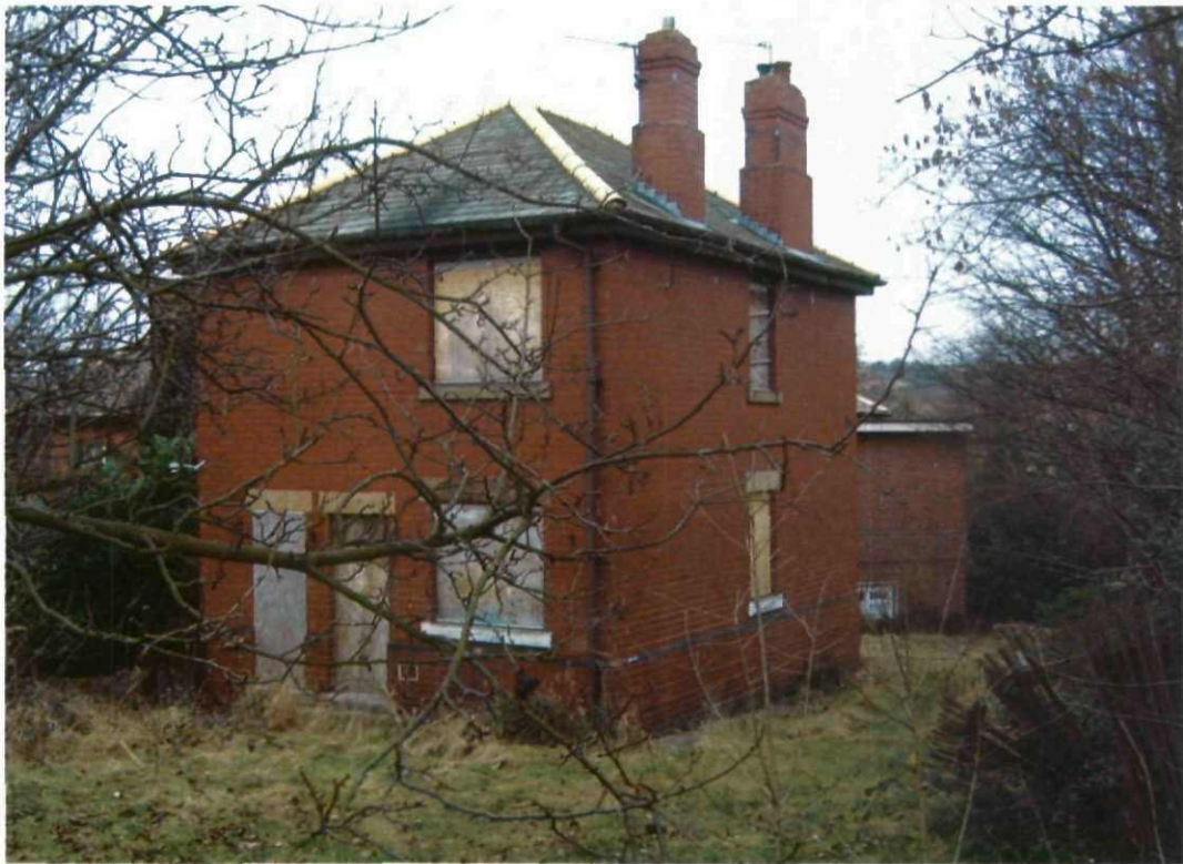
Plate 4 House on concrete platform to rear of council offices
