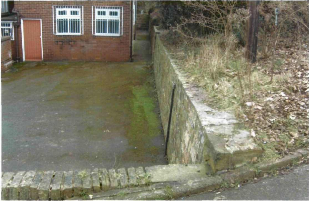
Plate 3 Revetted wall across middle of the site
