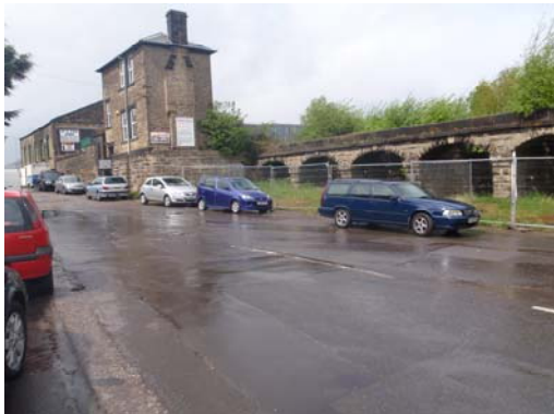
Photo 2.2 Existing Site (Eastern end near coal drops)
