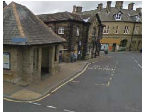
Photo 2.4 Existing bus stop Market Place
