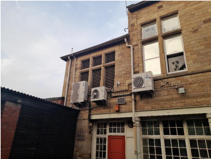
Figure 7 Louvre vents on western and northern elevations.
