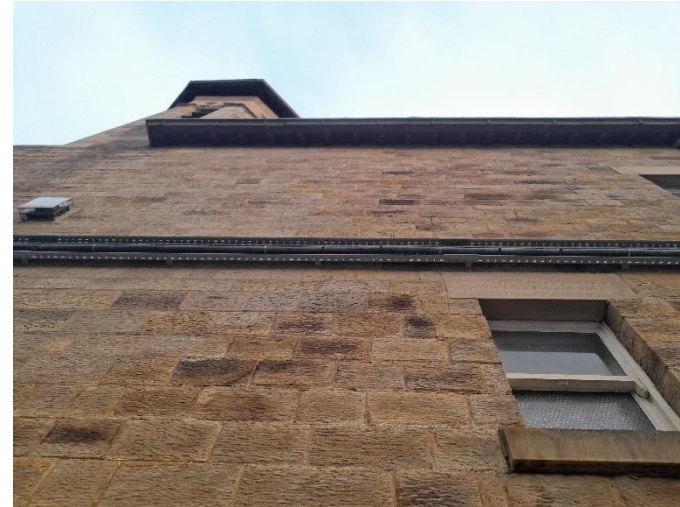
Figure 8 Duct and vented window on northern elevation.
