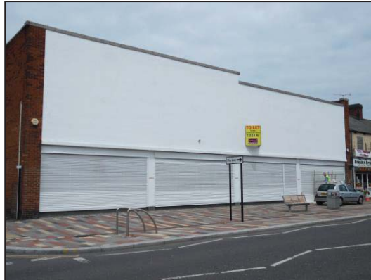
Image 4: Site viewed from Doncaster Road
