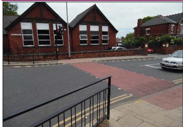
Image 6: Dropped kerbs creating inclusive access
