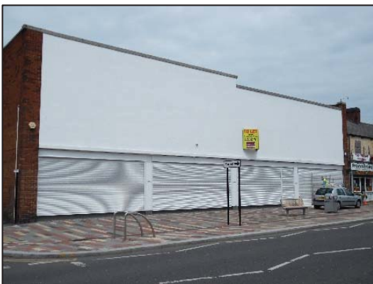
Image 1: Former 'Co-op', Doncaster Road
