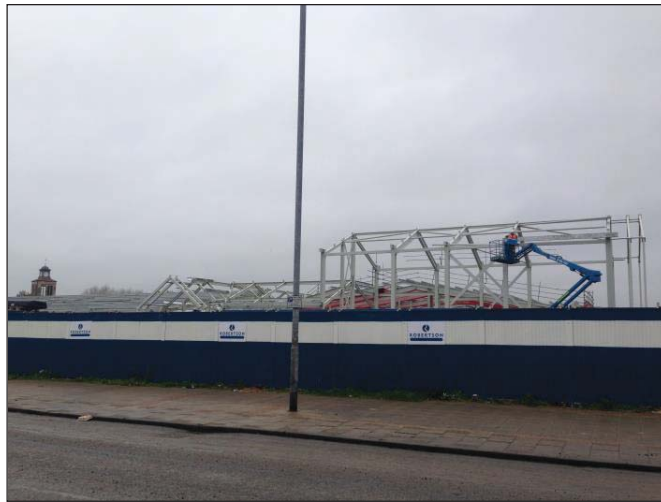
Image 2: Development Site viewed from Doncaster Road
