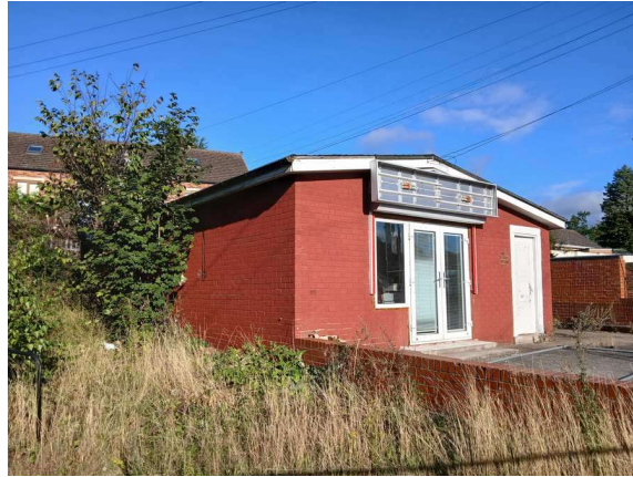
Building B1, facing north-west
