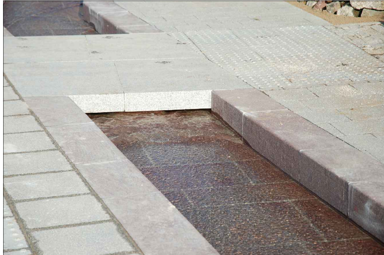
6 Paved crossing points with water underneath
