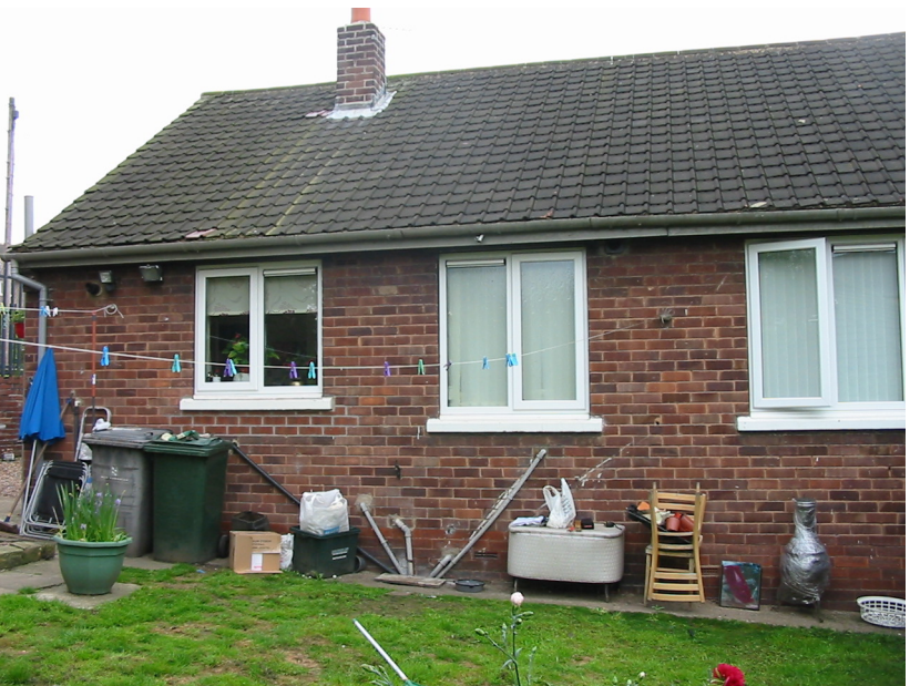
Existing view of rear of bungalow.
