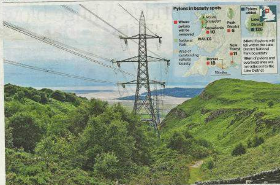
Electricity pylons in Snowdonia, one of four areas from which they will be taken away. There are plans, however, to install more than 120 in and around the Lake District
