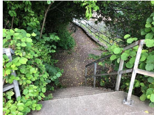
Existing Steps to Public Right of Way
