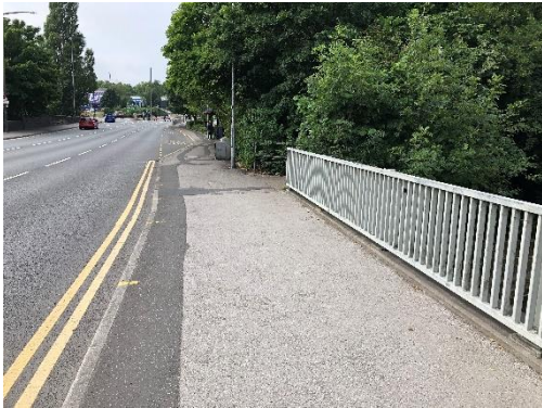
Old Mill Lane Bridge looking south
