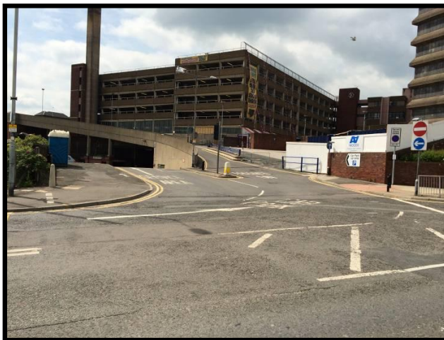
Photograph 1. Existing In-Only Access – Kendray Street
