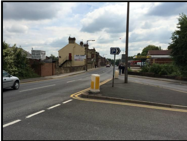
Photograph 4. Lambra Road / Pontefract Road Priority Junction
