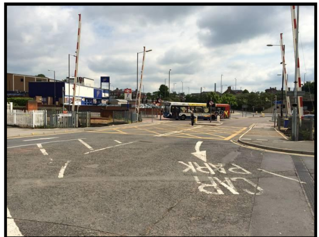
Photograph 2. Existing Kendray Street level crossing
