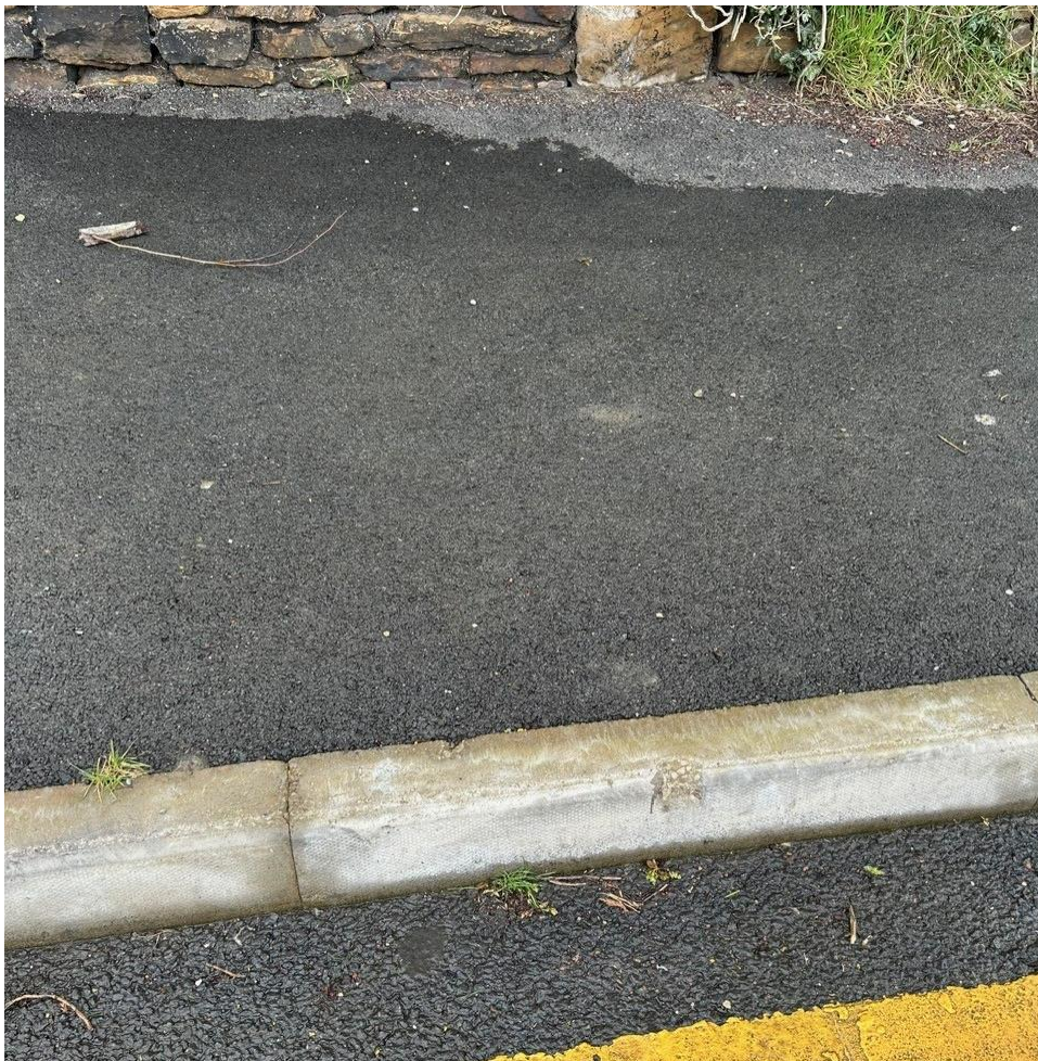
Image 3 – Damaged Kerb
