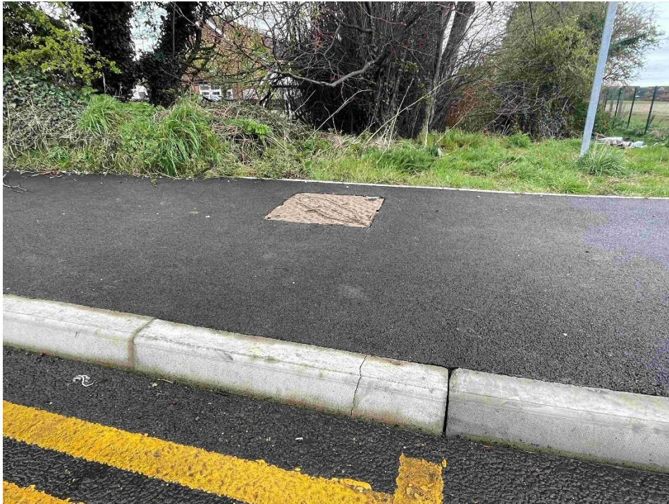
Image 2 – Cracked Kerb
