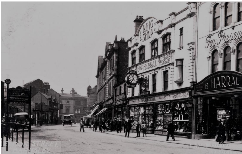
Fig 23. Historic photograph of the Harral Building from the 1920s showing the faience lettering to the arched pediment (reproduced with kind permission of Barnsley Archives).
