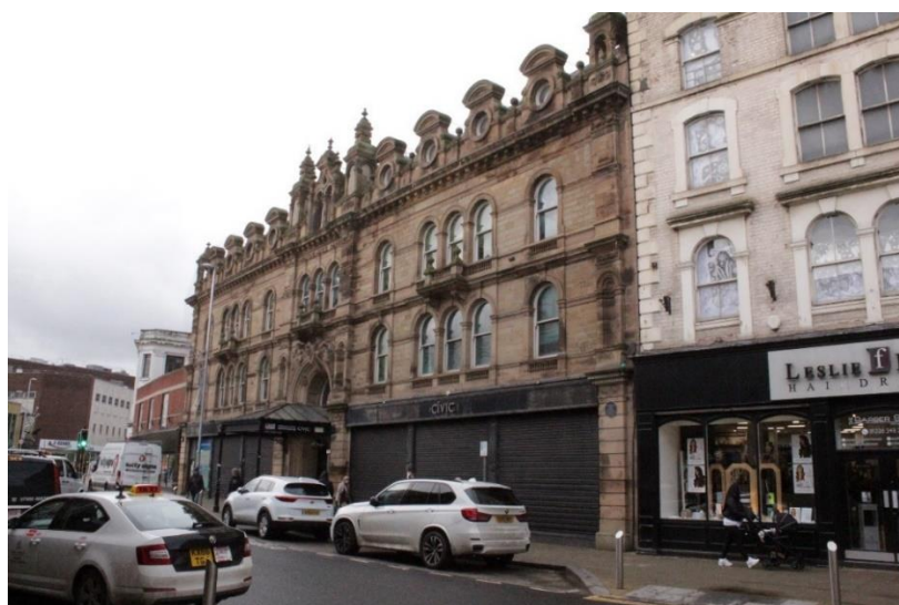
Fig 10. Eldon Street frontage of the Civic Theatre
