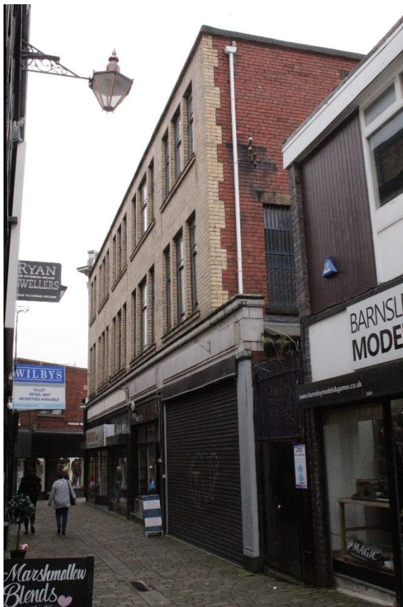
Fig 27. The Arcade elevation of the easternmost block (looking towards Eldon Street)
