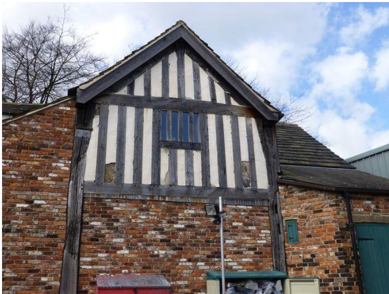
Fig 12. Close-studded gable of 41-43 Church Street
