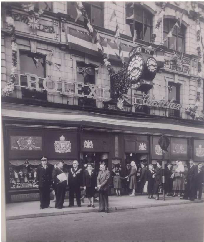
Fig 22. Photograph of the Harral Building on the 29 th May 1953 (Barnsley Archives).
