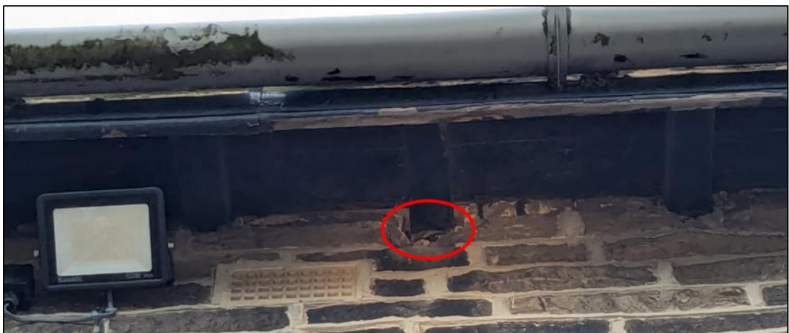
Plate 17. Gap between protruding rafter and masonry
