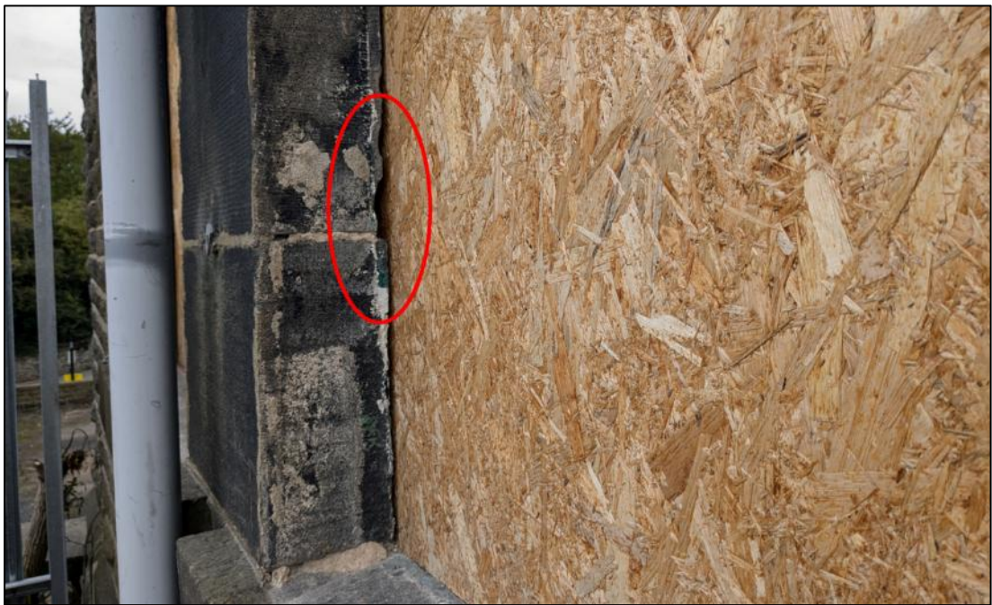
Plate 17. Gap between protruding rafter and masonry
