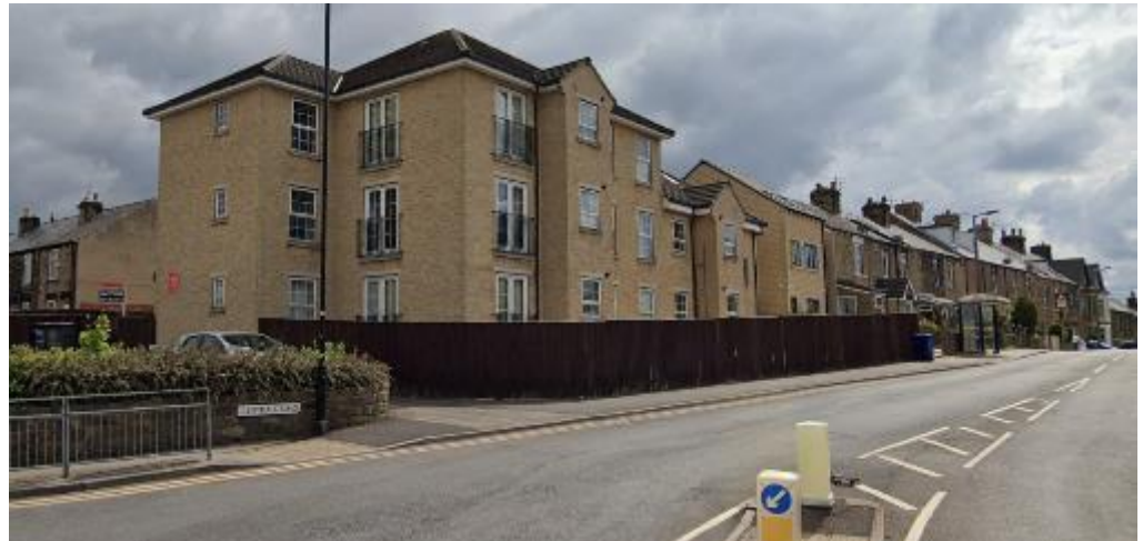
New row Court Flats seen from Barnsley Road and no more than 75 metres from the Application site are 3 Storey and of simple design
