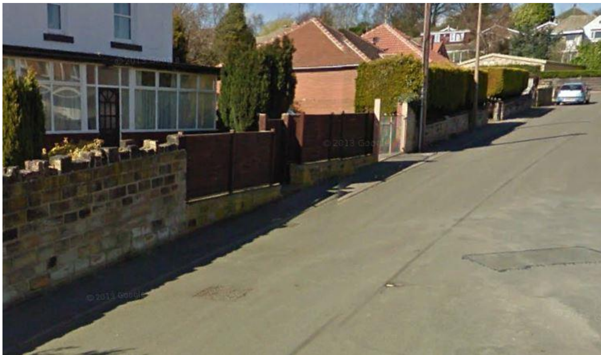
STONE WALL AND TIMBER FENCE ON VICAR ROAD
