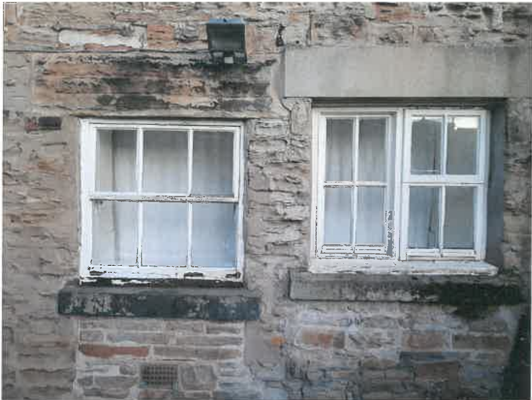
Figure 4 – Existing ground floor rear elevation windows
