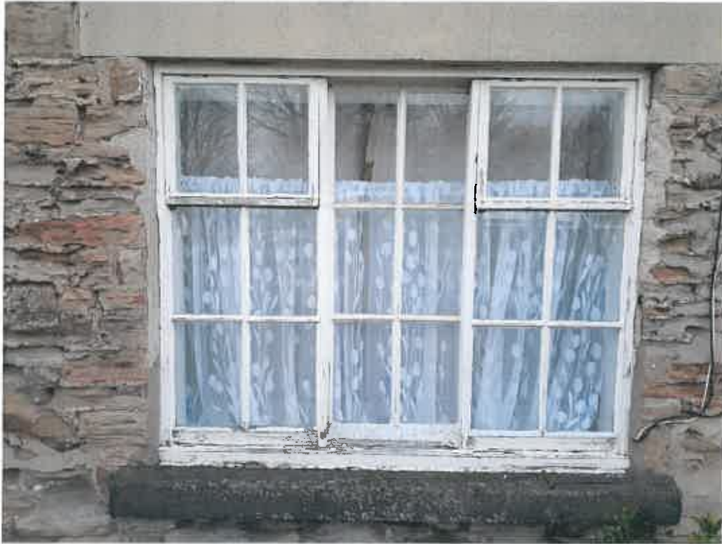
Figure 3 – Existing ground floor front window
