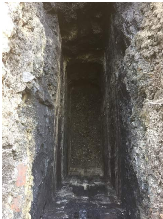
TP11 – Made ground over coal separated by dirt bands.
