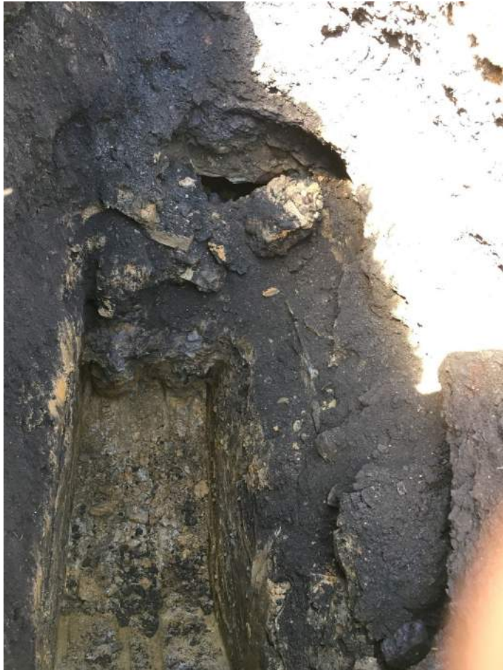
TP1 – Made ground over natural clay from 1.6 m
