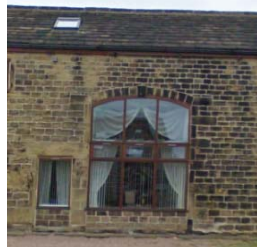
Thursltone barn conversion with large glazed barn door
