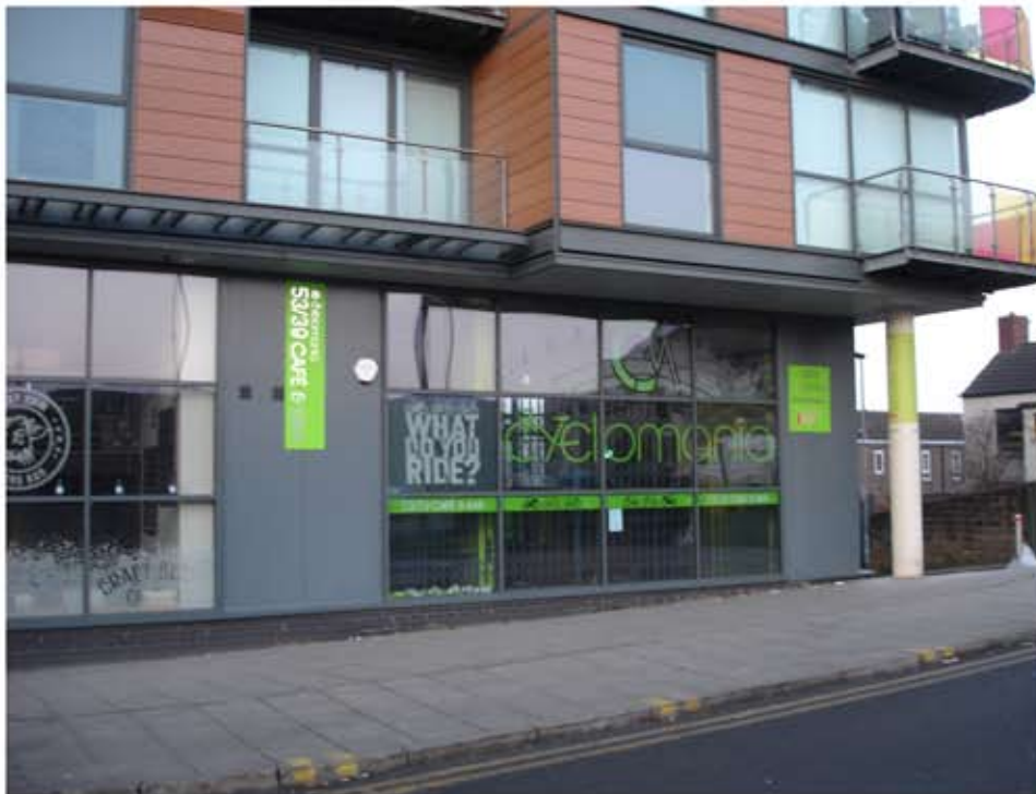
Existing Shop Front
