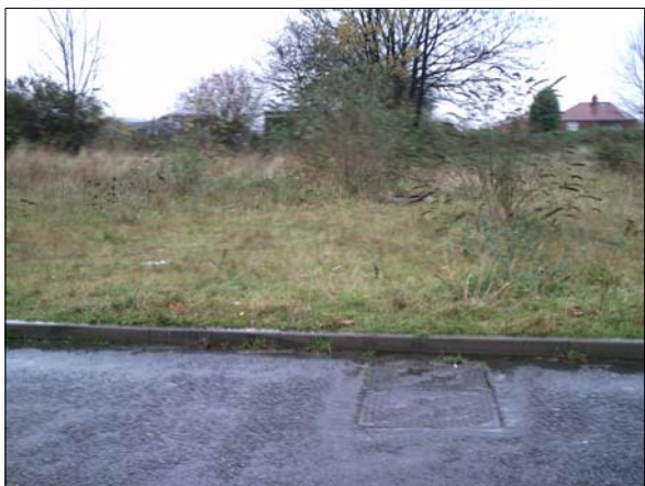
Title: GP7 Date: 21/11/12 Description: PUBLIC MANHOLES 1 - LOCATION
