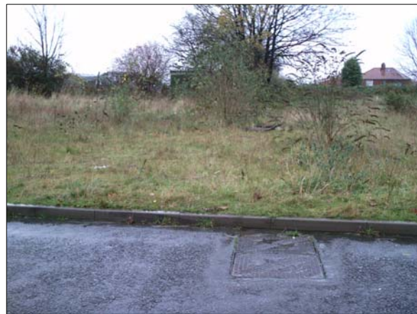
Title: GP6 Date: 21/11/12 Description: PUBLIC MANHOLE 1 - LOCATION
