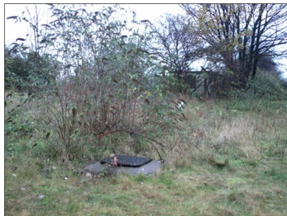
Title: GP8 Date: 21/11/12 Description: PUBLIC MANHOLE 2 - LOCATION
