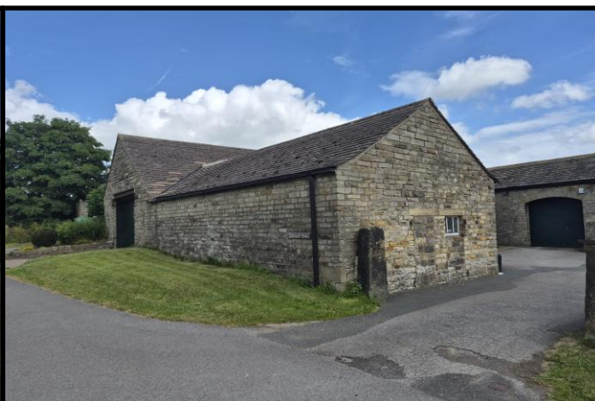
Photograph 2. Barn from road
