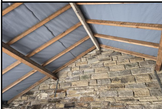
Photograph 3. Internal of Barn
