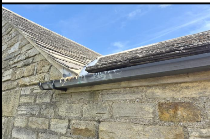
Photograph 6. Example of roof and tiles
