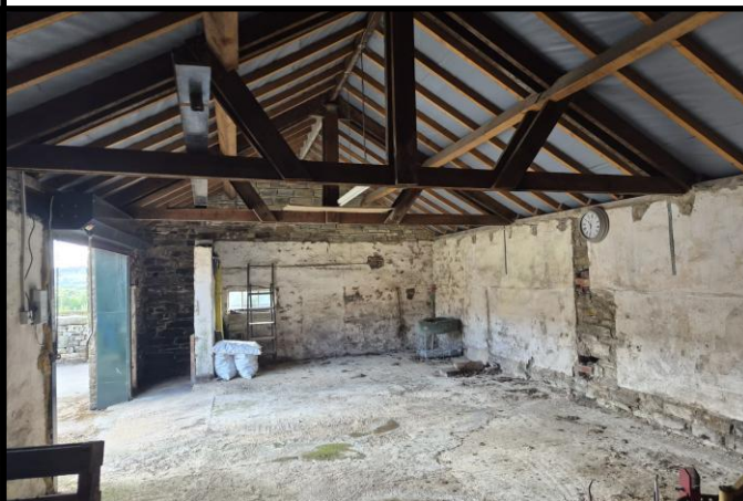
Photograph 4. Internal of Barn
