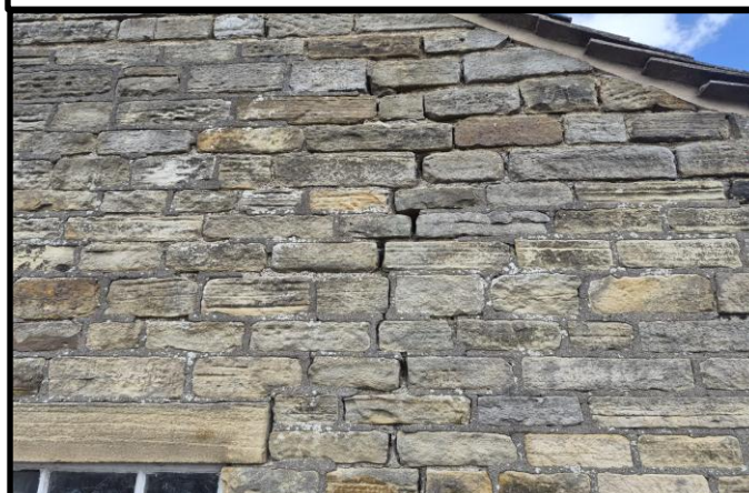
Photograph 5. Example of external crevices
