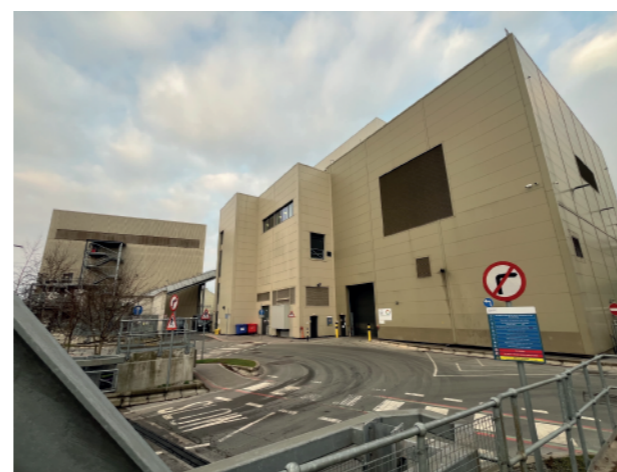
Example of exterior painting system used by SRC at The Templeborough Biomass CHP Facility in Rotherham.
