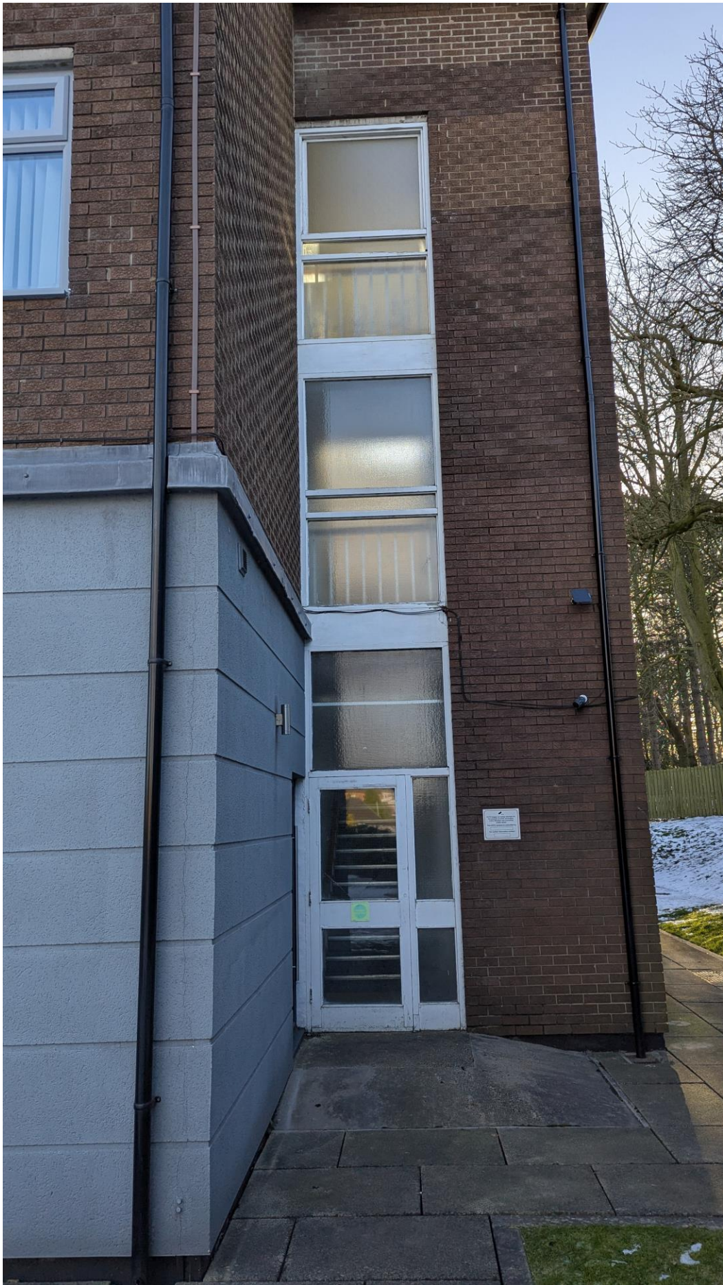
Photograph of exterior of window/door to fire escape Stairwell
