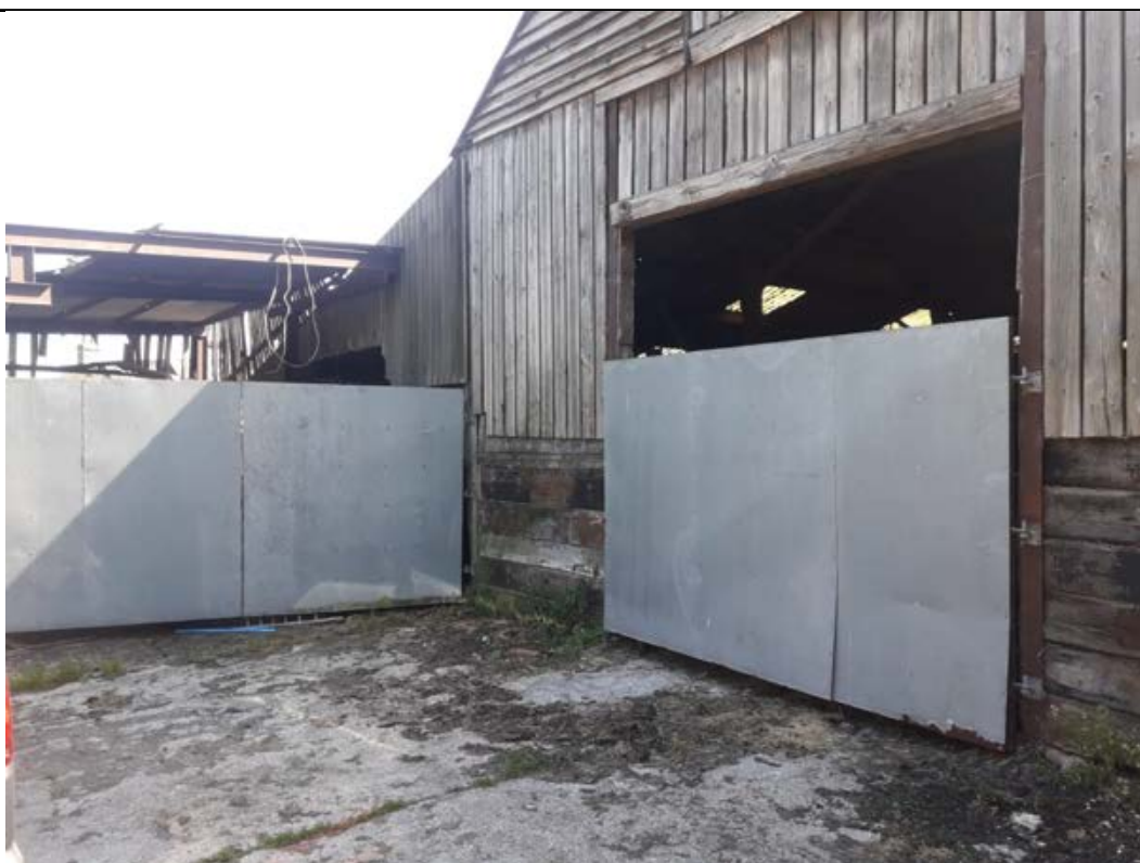
North-eastern corner (Facing west).
