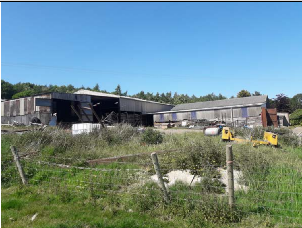
South-east corner facing north.
