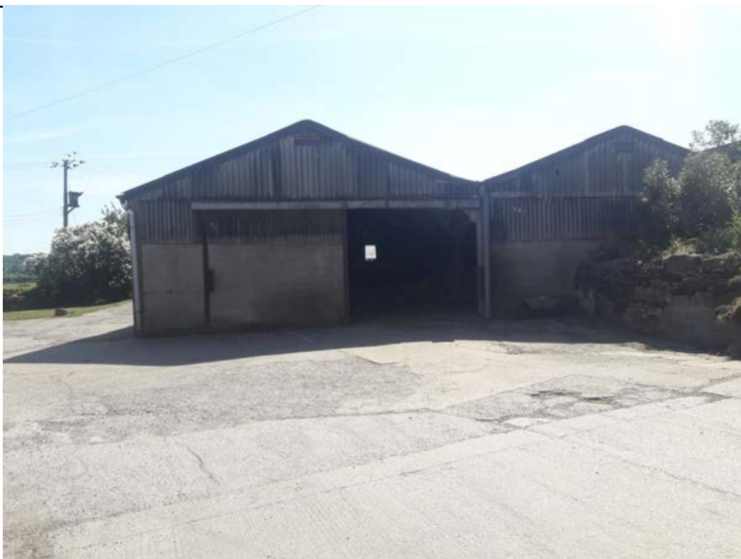
Southeast area (Facing east)
