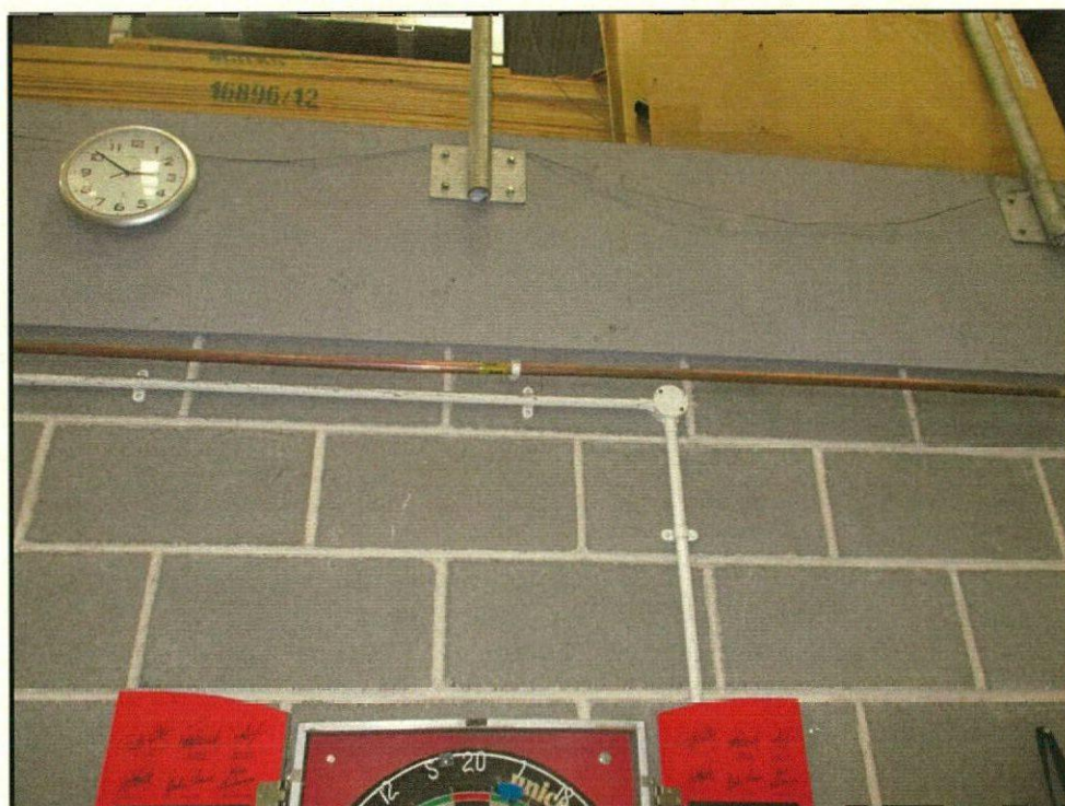
Photograph 14 Unit 20 interior; minor alterations to gas and electricity supplies may be necessary.
