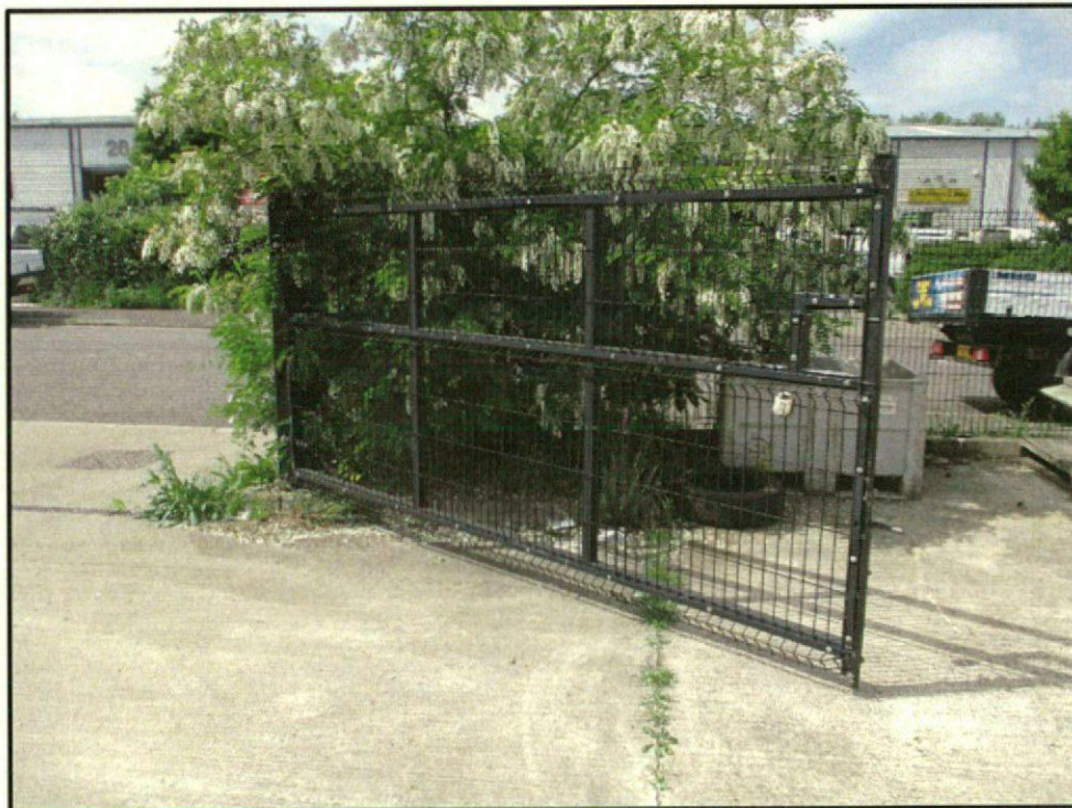
Photograph 4 Units 20 & 21 shared access security gate.
