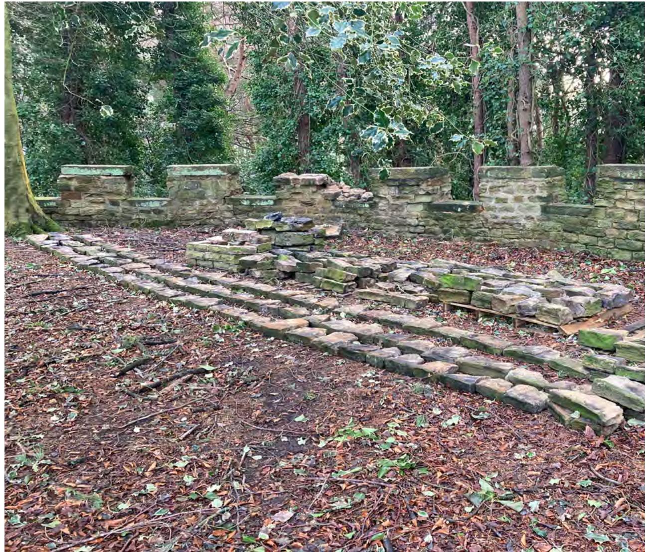
Sorting of Existing Stonework
