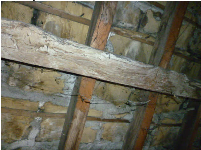
Photo 2: Cement torching in main roof
