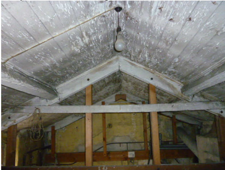
Photo 3: Wooden sarking lining roofing slabs
