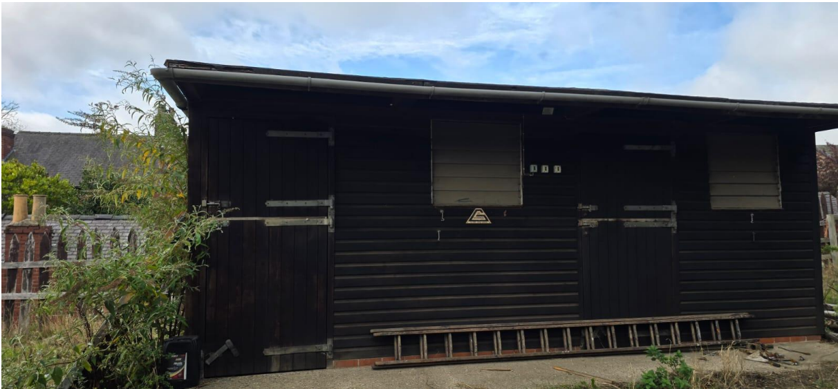
Photograph 3: General view of site
