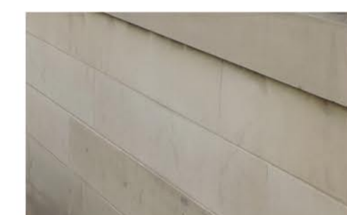
York Stone on building opposite to be used to match stone on new wall.
