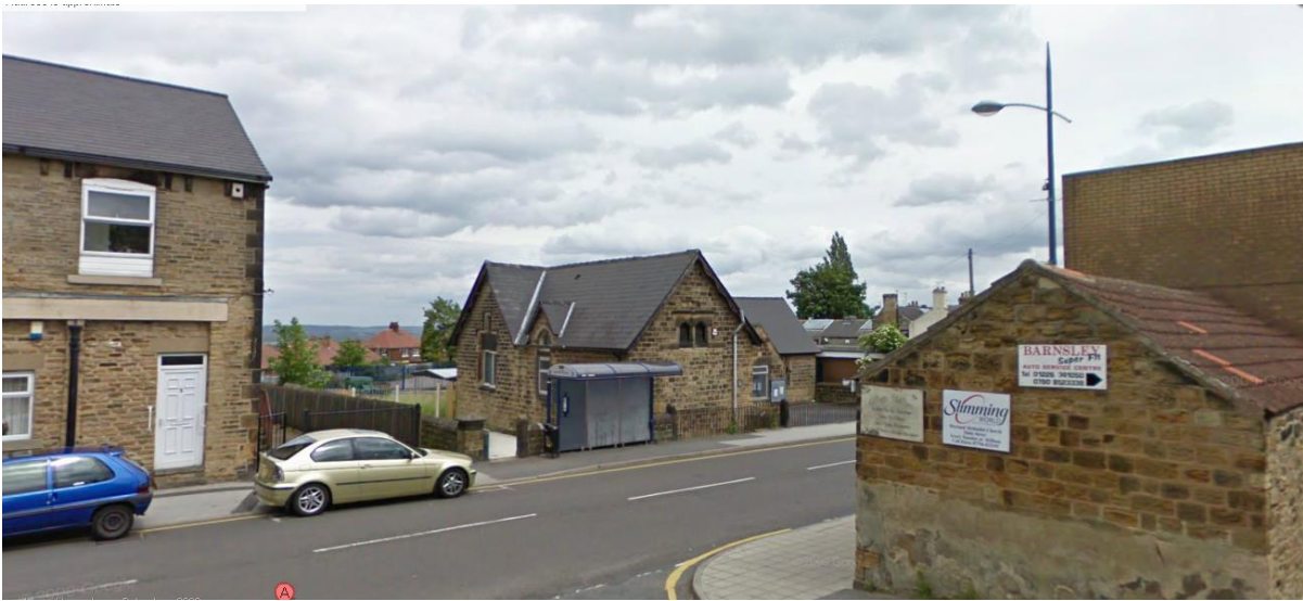
VIEW FROM OPPOSITE SIDE OF MARKET STREET
