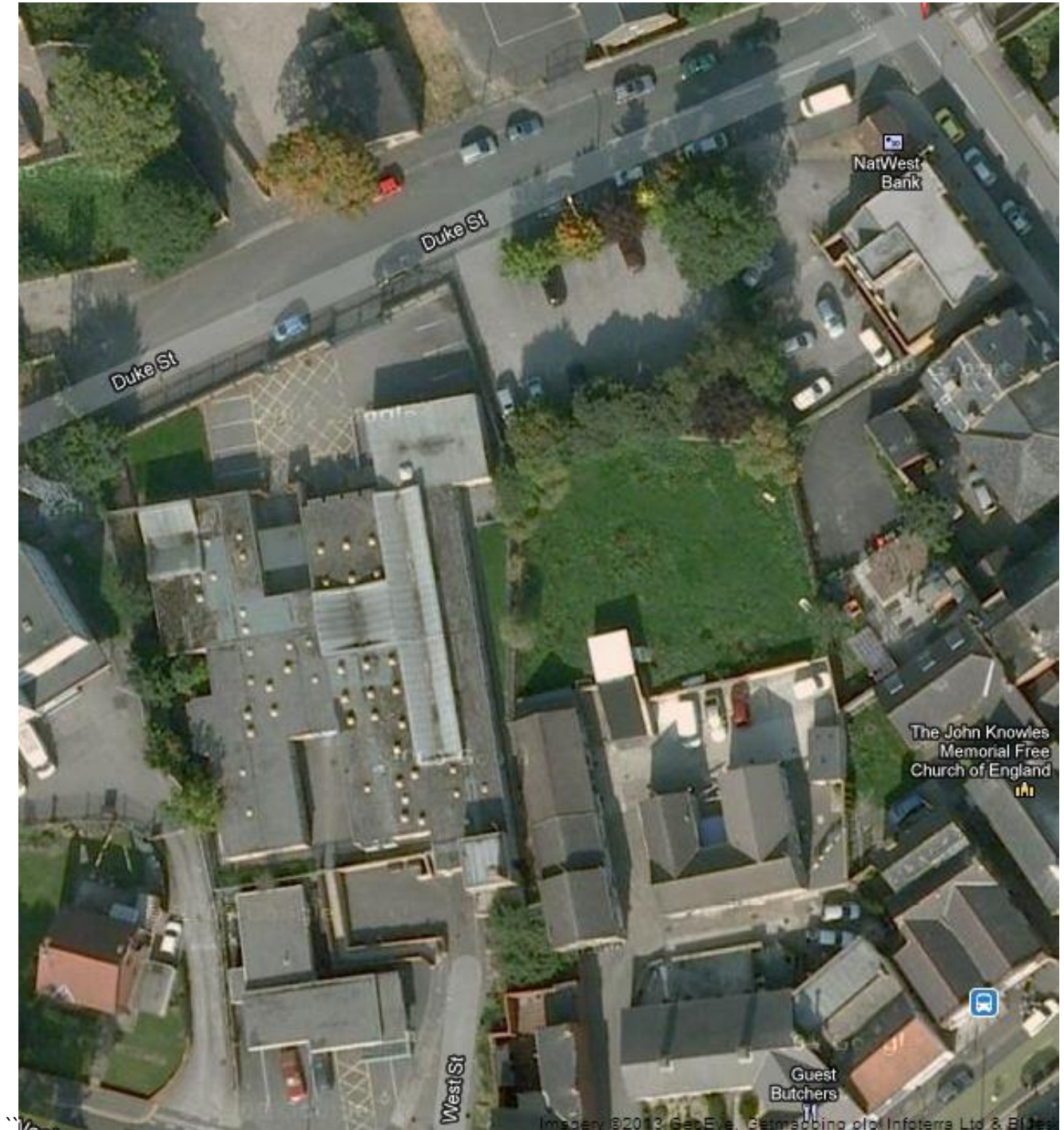
SITE A AERIAL PHOTOGRAPH
