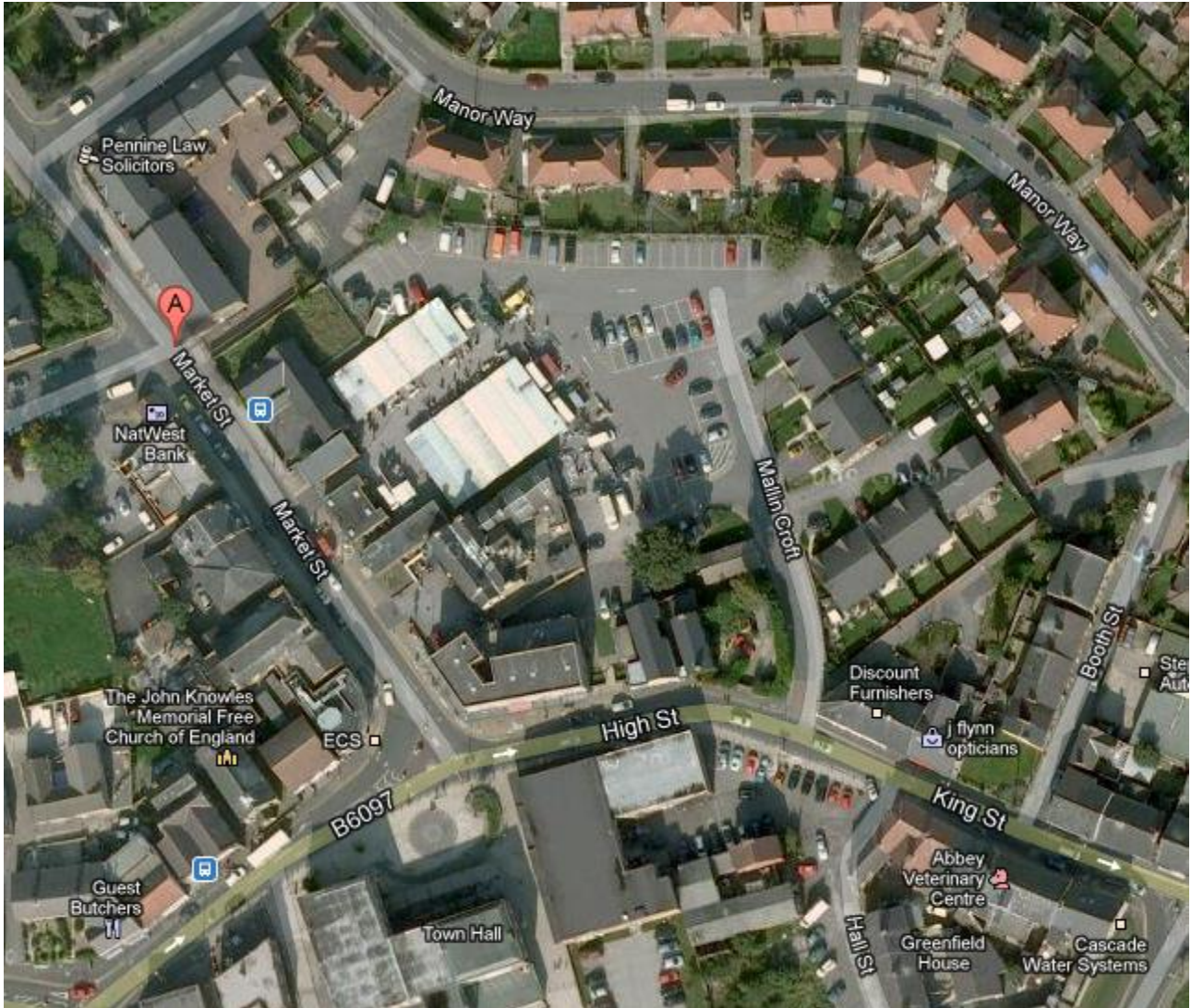
SITE B AERIAL PHOTOGRAPH
