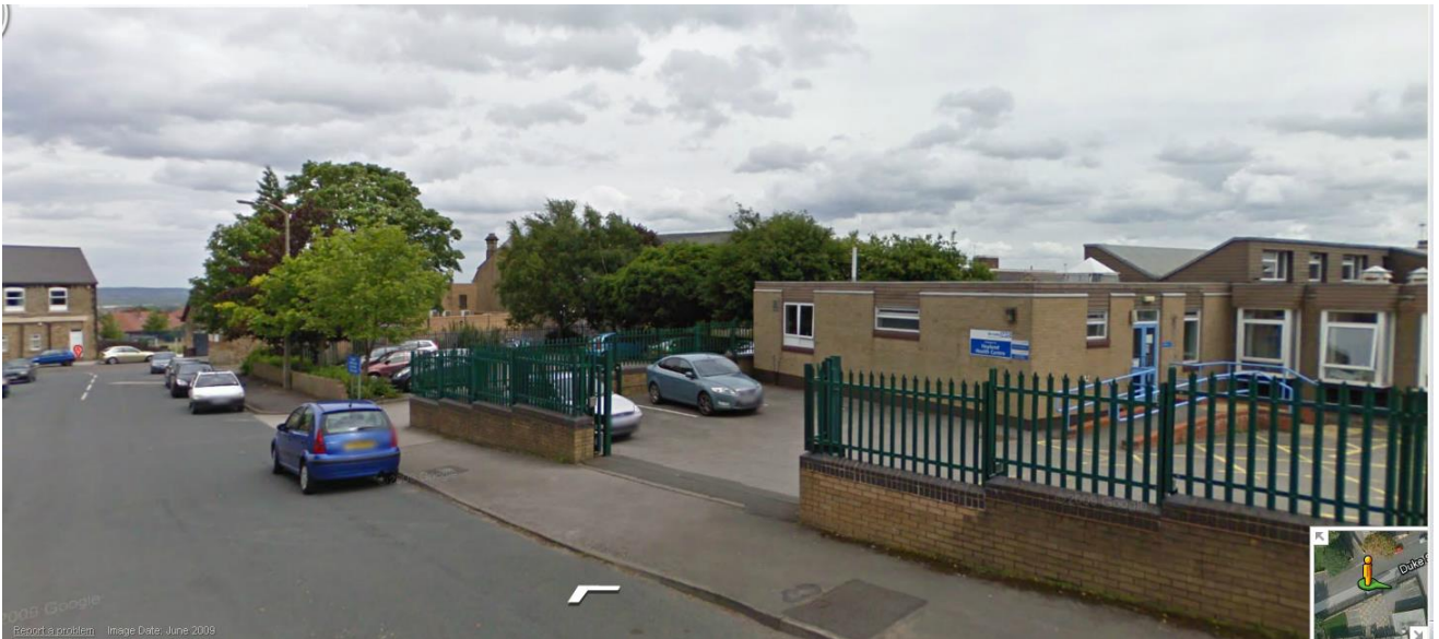
VIEW FROM DUKE STREET
