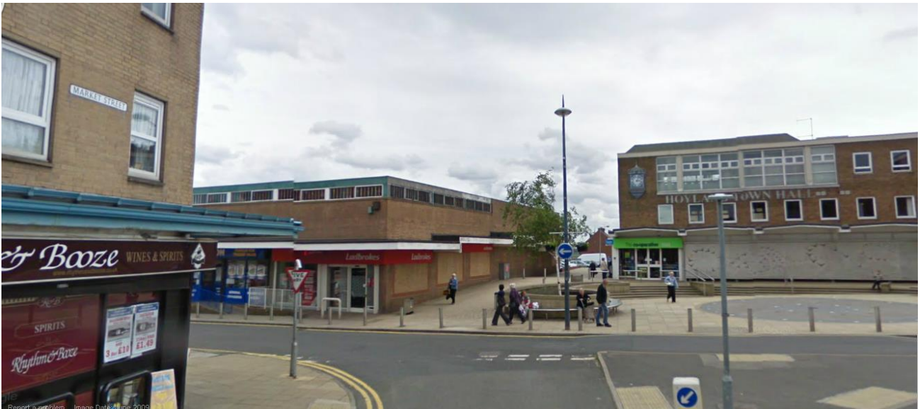
VIEW TOWARDS MARKET STREET/ HIGH STREET JUNCTION
