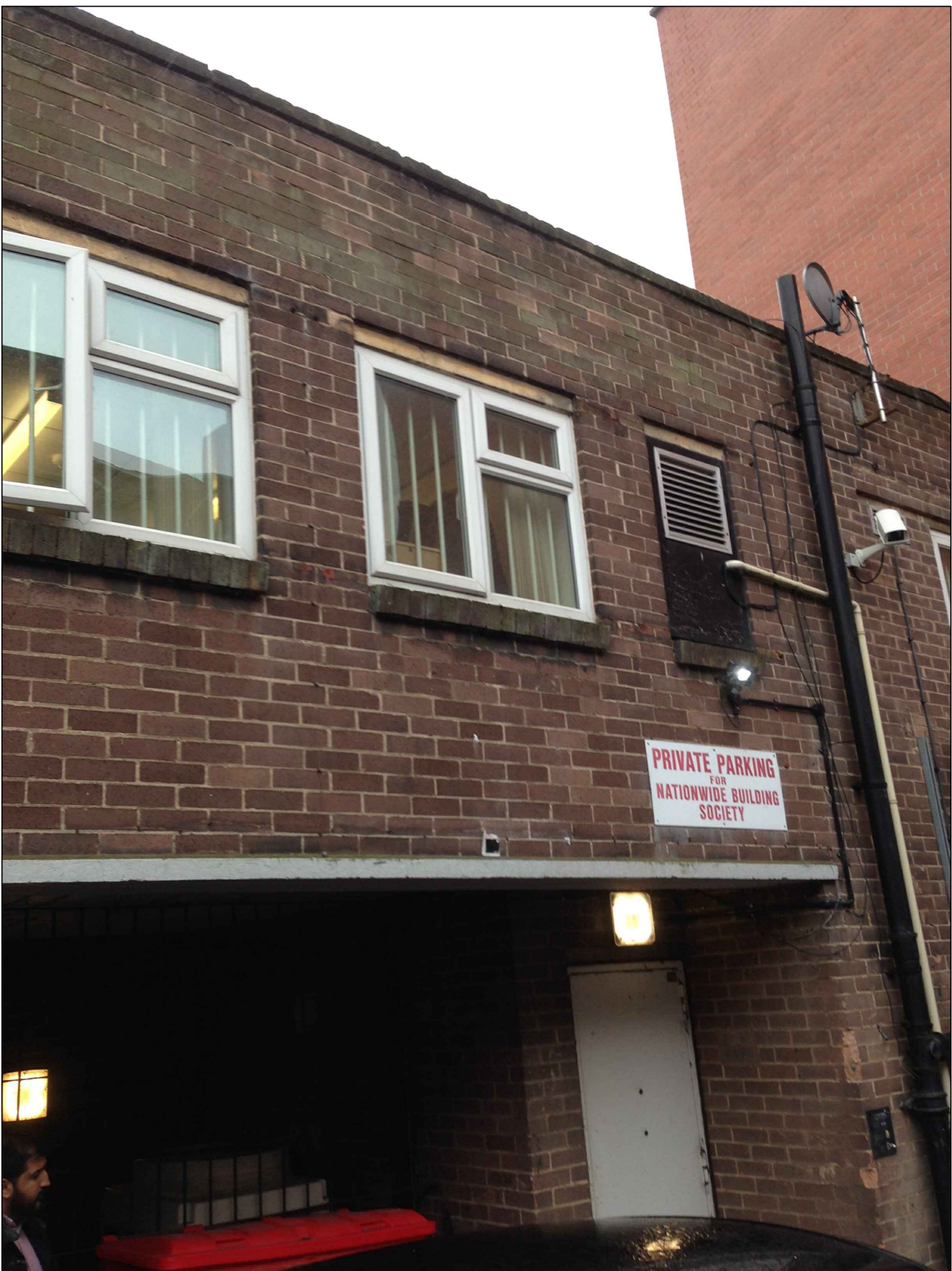
SITE PHOTO | EXISTING LOUVRE
