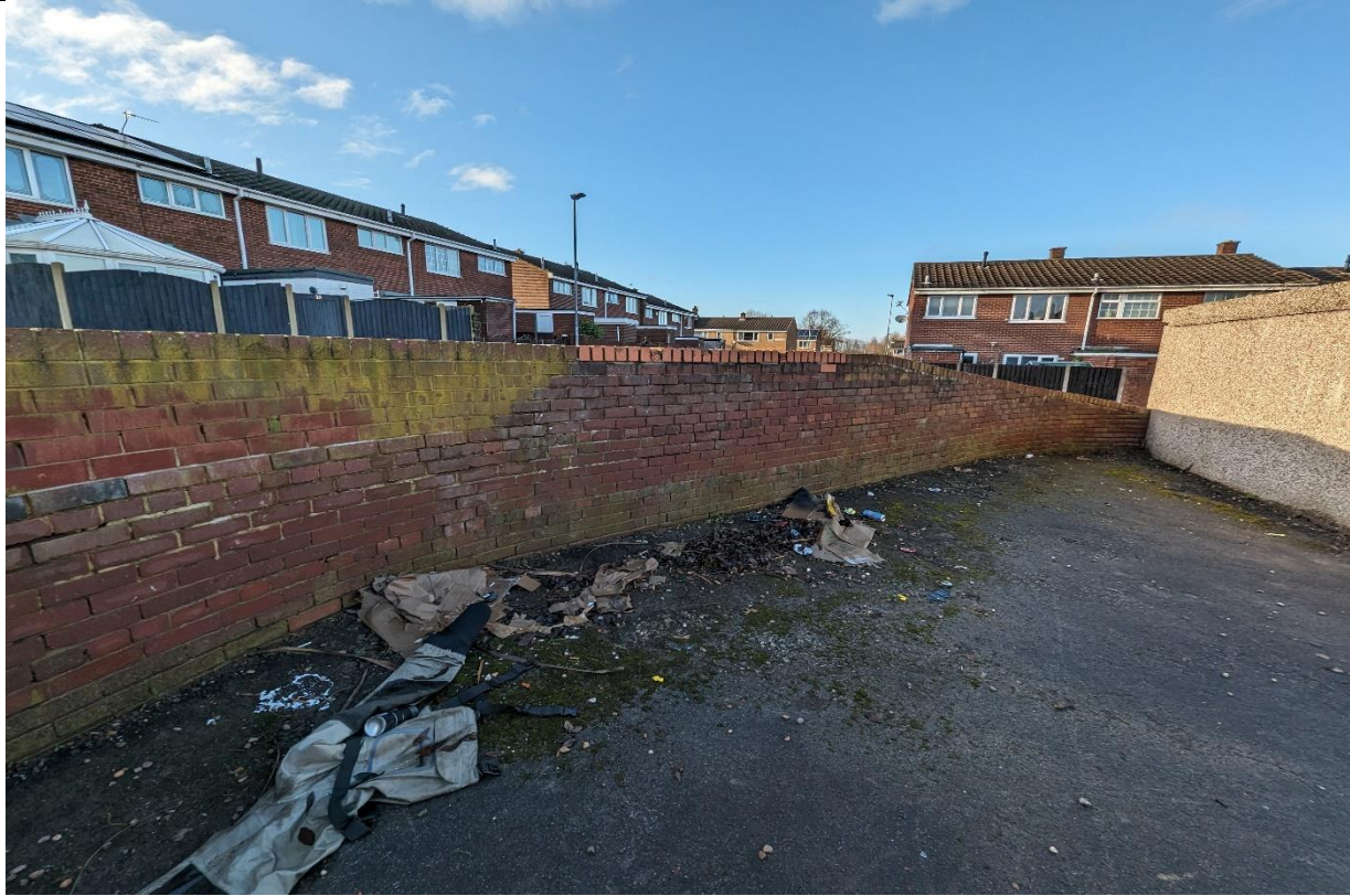
Photo 3 – View on Low side of wall
