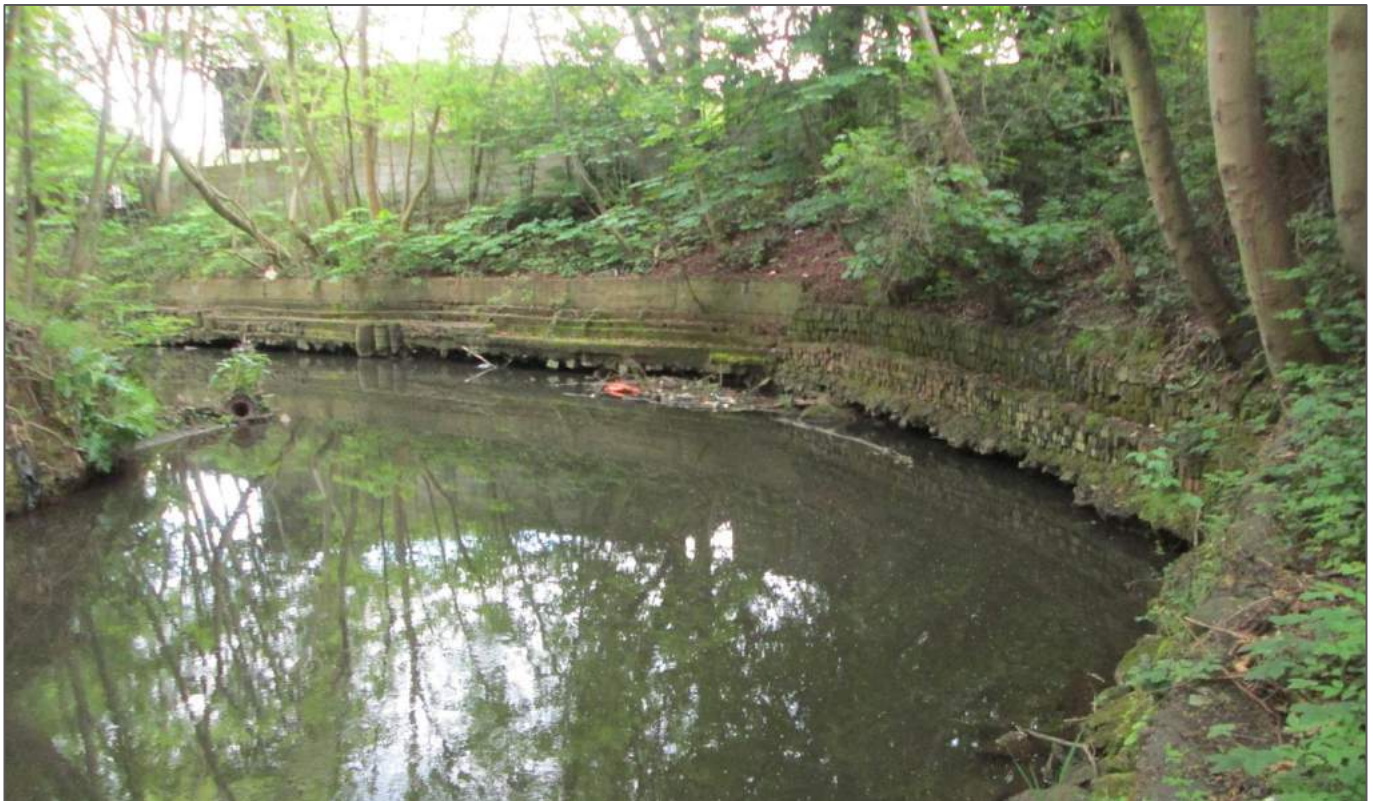
Plate 3: Section of the River Dearne which lies to the north of the site.
