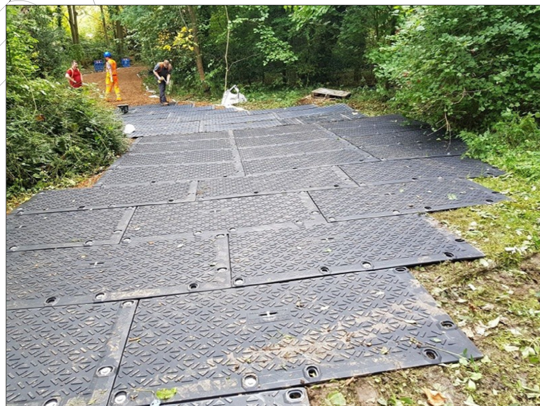
Ground protection boards
