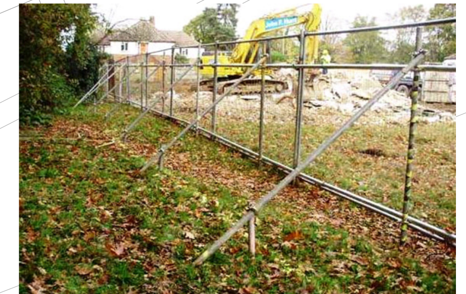
BS 5837:2012 tree protection fencing
