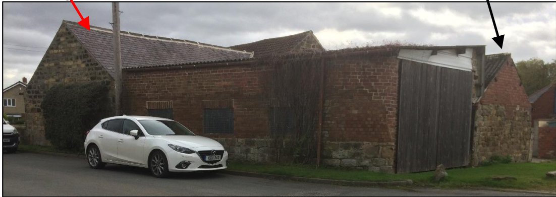
Plate 8. Example of roost potential in external walls of stone barn
